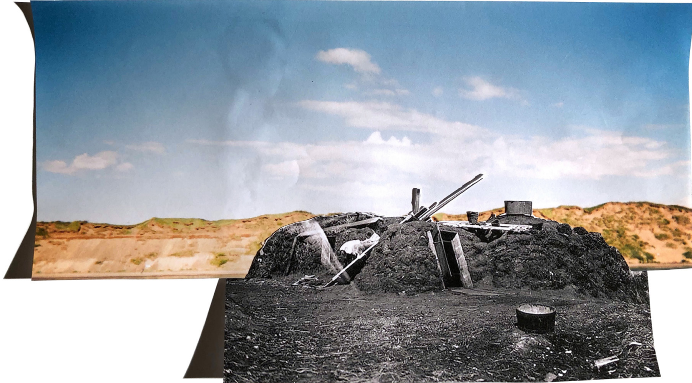
A barabara, a half-pit sod home, made from bluffs along the shore.
