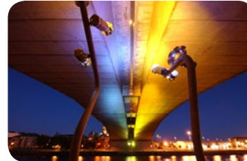
Figure 6-111. Colored lighting washes on structures. Chroma Streams, Kingston Bridge, 2005 by Leni Schwendinger. Photo courtesy of lightprojectsLtd.com
