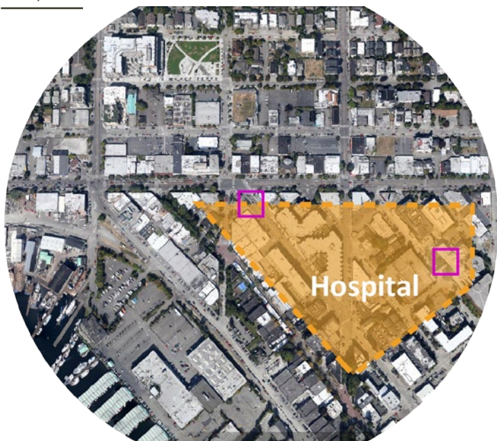
Figure 5-72. Hospital subdistrict. Location of hospital emergency entrance and Bergen Plaza marked by the squares.
