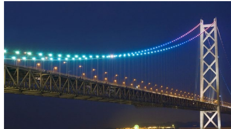
Figure 1-23. Pearls of Light, Akashi Kaikyo Bridge, Kobe. Photo courtesy of listofimages.com
