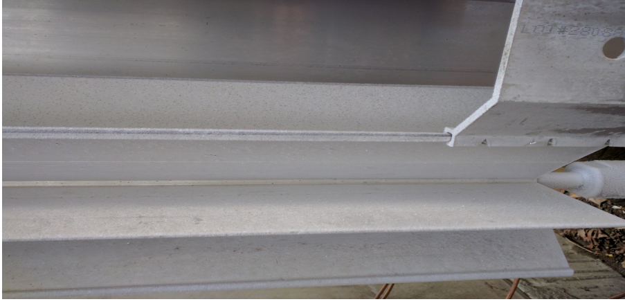
(c) Close up of the frost formation.
