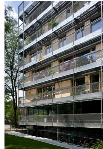
Figure 19: R50 Exterior | Source: Andrew Alberts
