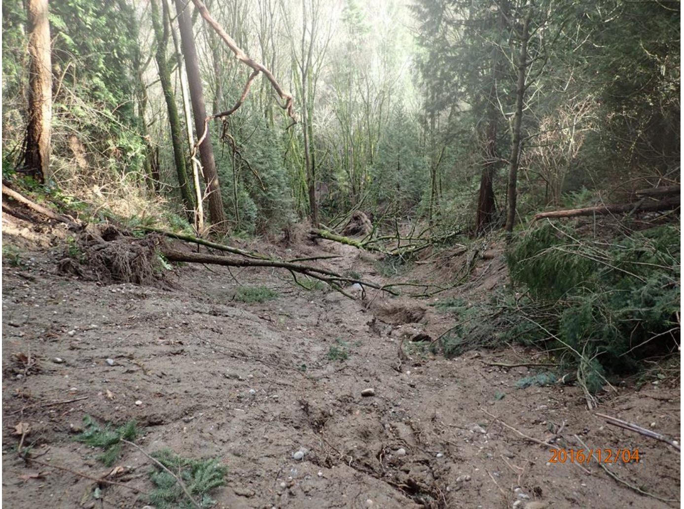
Figure 20: Photograph of scour and debris resulting from a shallow landslide that occurred in the Finn Hill area near the end of November.
