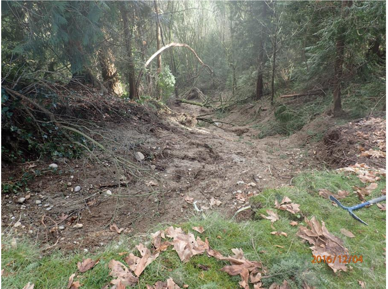
Figure 19: A photograph of the initiation point of a recent shallow landslide in the Finn Hill area. The slide uprooted and carried mature trees. It also ran up the opposite valley wall approximately 50 feet. The pick end of my geotool is fourteen inches long. See Figure 21 for slide location. The recent slide exists within an area of historic landslides.
