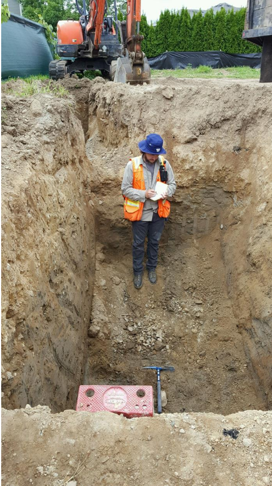
Figure 10: The author making observations at a construction excavation in Vashon Till (Qvt).
