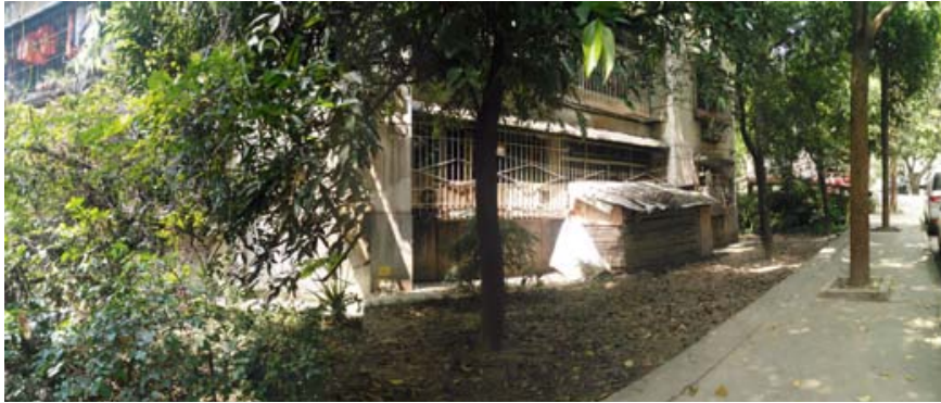
Figure 4.51. Old secondary neighborhood street's existing photo 1
