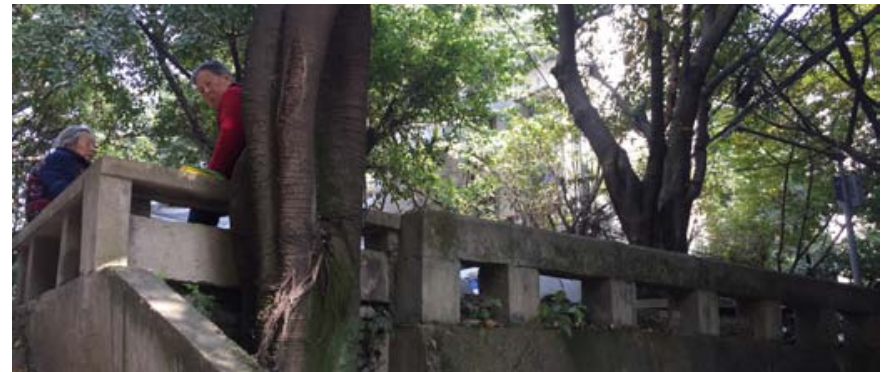
Figure 3.14. The retaining wall and fencing wall in the old areas
