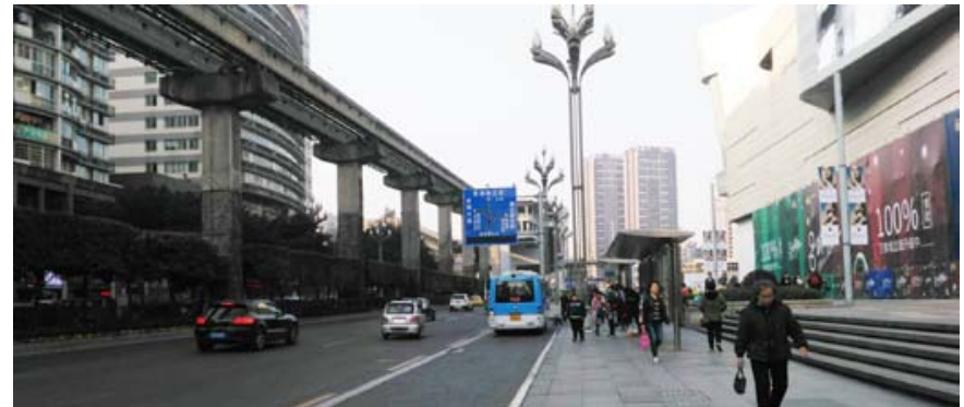
Figure 3.41. The bus-stop in the new area
