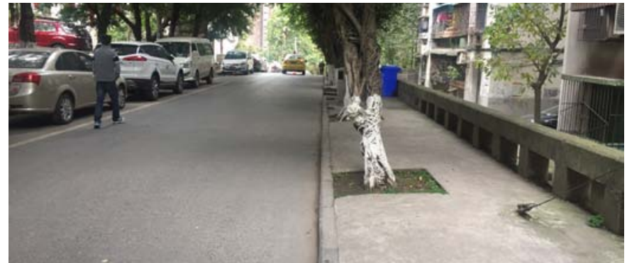
Figure 3.27. The lack of grates for trees in the old area
