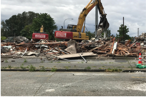
10. Demolition of Montlake market. Seattle 2020
