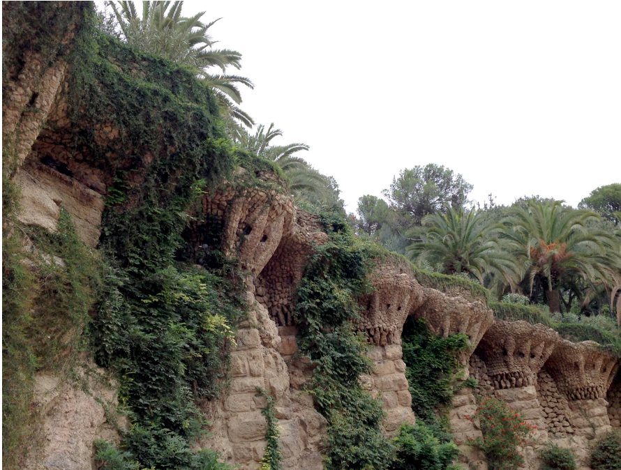
1. Large vernacular retaining structure, Park Güell
