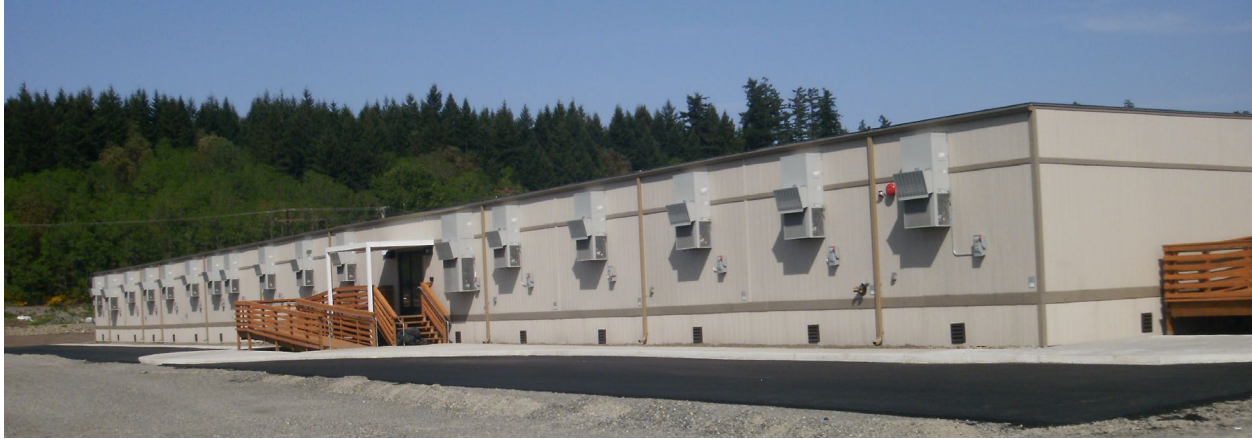
Figure 1.3. 30,870 square foot re-locatable modular facility | Photo by SMM
