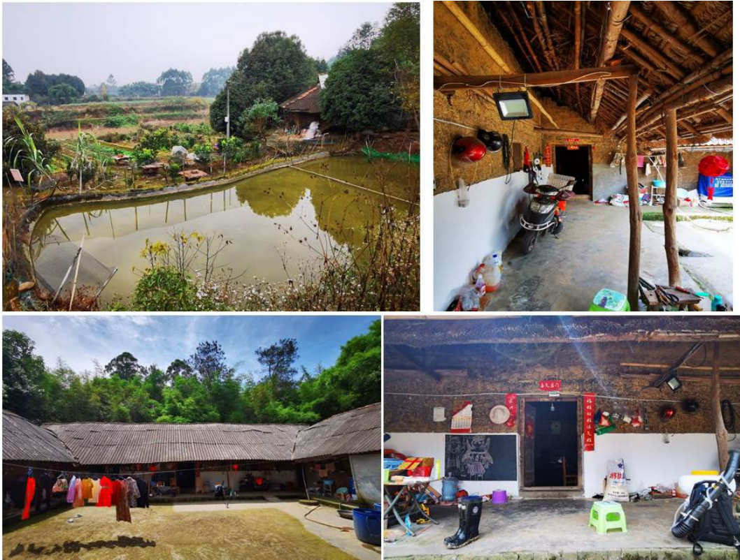
Figure 2.19 Environment and house of the “U” shaped settlement owned by Zhou’s family Note: Top left: Farmhouse covered by tree and bamboo groves with water pond and farming fields nearby; Top right: A wide porch in the front of main building, with view of mud wall, thatched roof and wooden pillars; Bottom left: “U” shaped settlement with main building at the middle and two wings on both sides; thatched roof being covered with asbestos tiles; Bottom right: Door to main room, viewing porch as a public space
