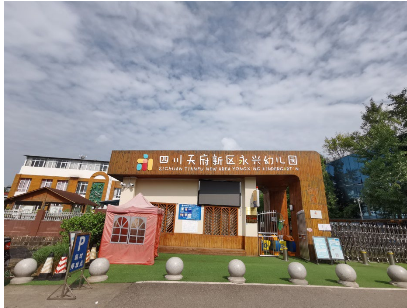
Figure 3.35 A newly established kindergarten at Yongxing Zhen
