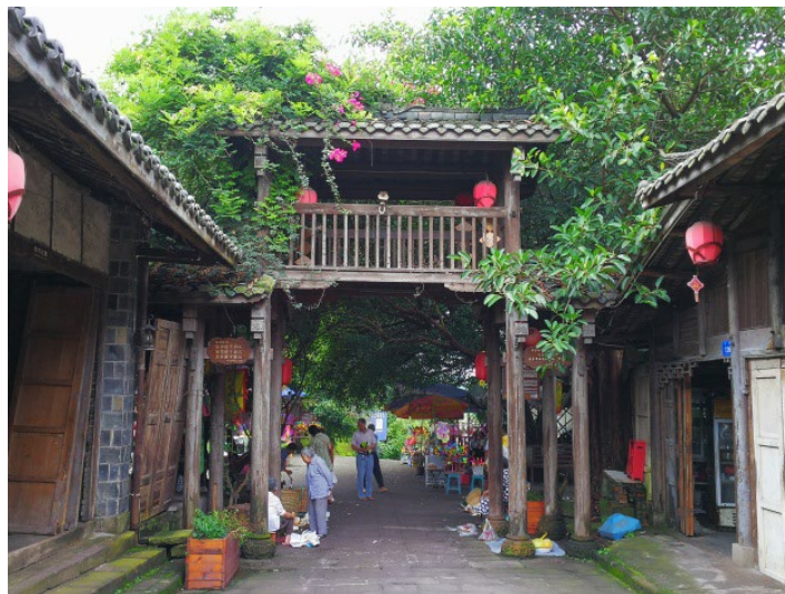
Figure 3.12 A traditional town gate with wooden framework in Xianshi Town, Sichuan
