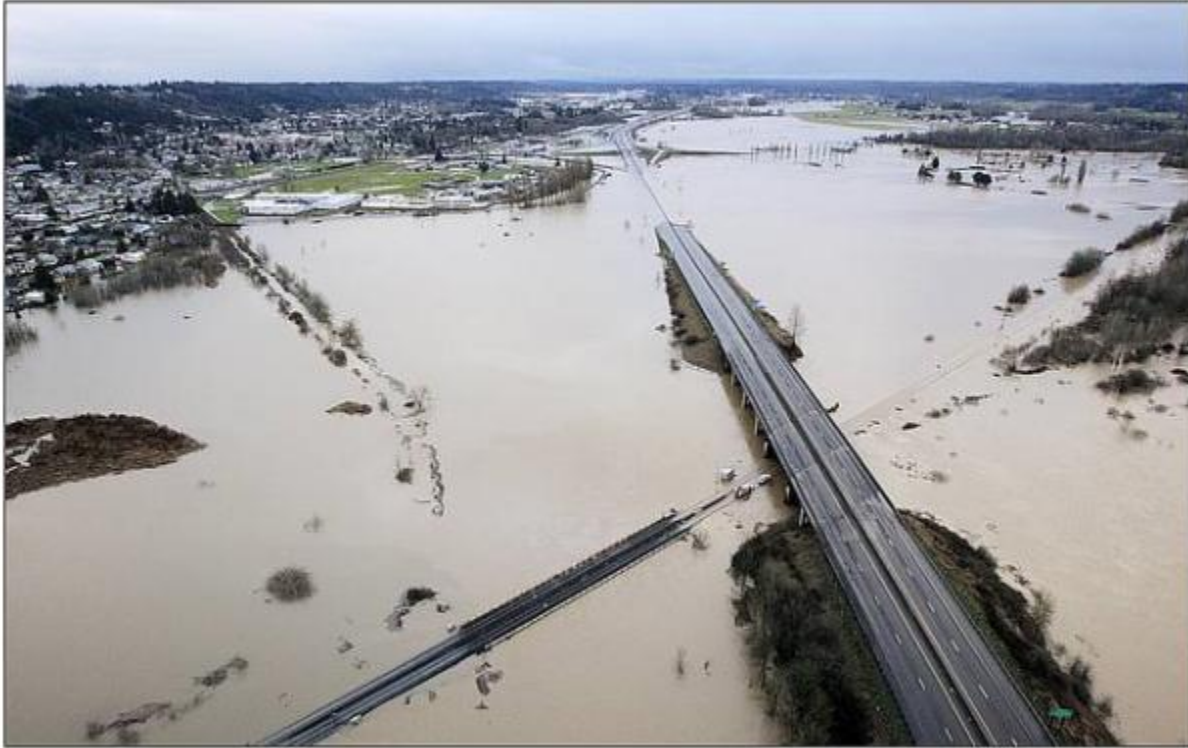
Flooding on Interstate 5 near Chehalis, WA on Jan 8, 2009. (Source: SeattlePI.com)
