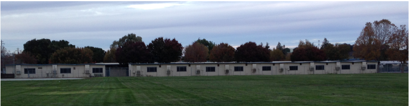
figure 29 : view of R.O. Hardin's existing portable classrooms from the south
