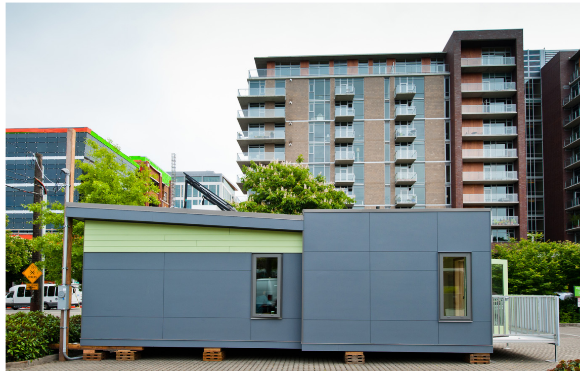
figure 12: exterior of the SEED Classroom
