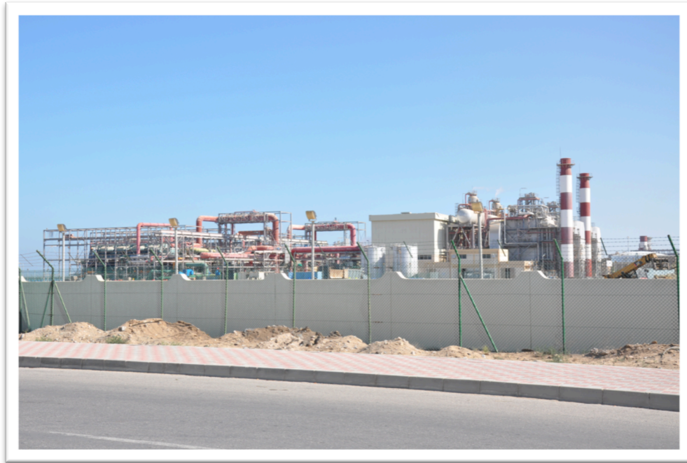
Figure 6: Al Ghubrah Desalination Plant
