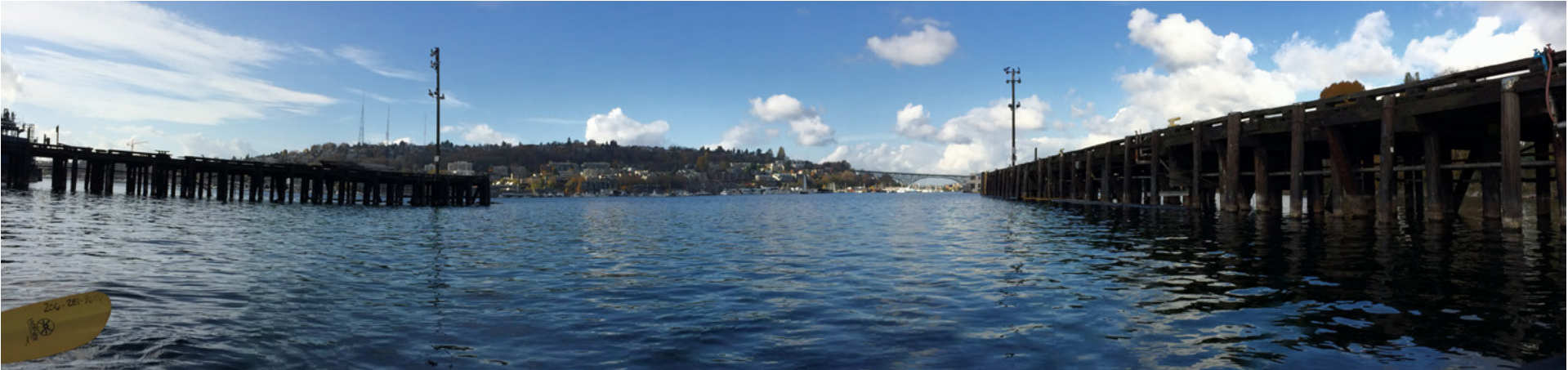
Figure 20. View looking west, between the two piers.
