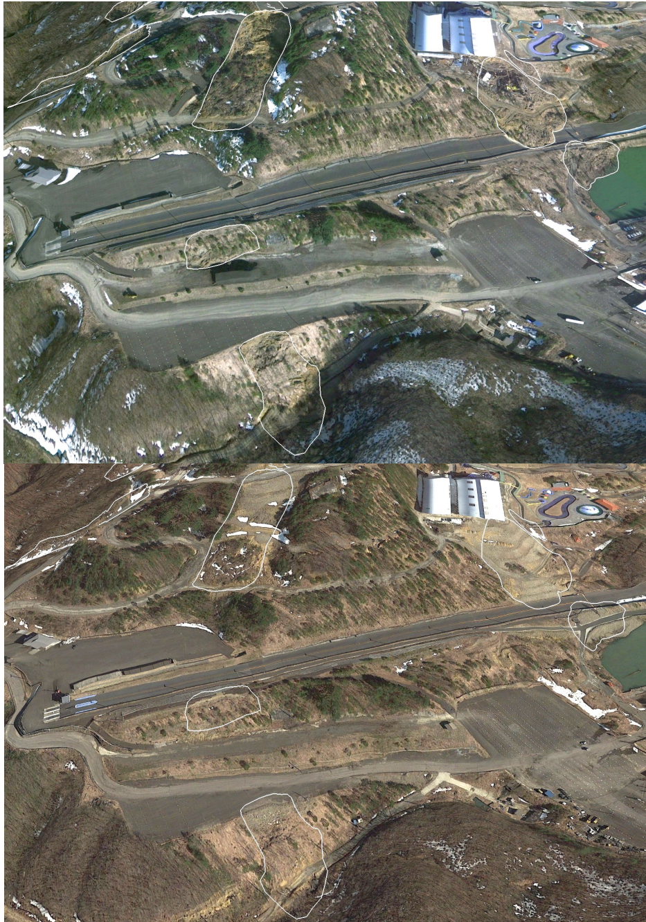
Figure 2.4 Landslides were mapped from the top image collected three weeks after the Tohoku earthquake. In many cases, these damaging landslides have been erased from the landscape (e.g., landslides on the right of the lower image, taken in 2014.) In many instances of smaller landslides, such as lateral spreads, evidence of landslide occurrence was completely erased from the landscape within months of the earthquake.
