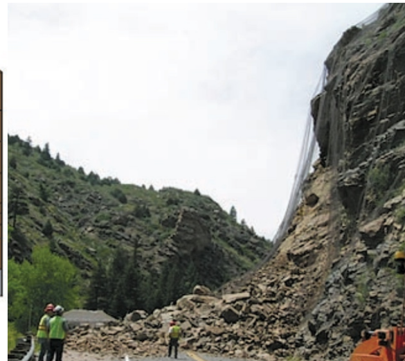
Figure 2.8 Simplified diagram (left) and an example Rock Irregular Slide. Diverse in failure mechanism, all involving large rock masses (boulders pictured are 8 – 10m long) failing from exposed bedrock. Distinguished from debris slides by the size of failed material (>5m blocks) and sense of movement including all falls and topples of intact material. Figure from Highland and Bobrowsky (2008), based on Cruden and Varnes (1996), photograph by the Colorado Geological Survey.
