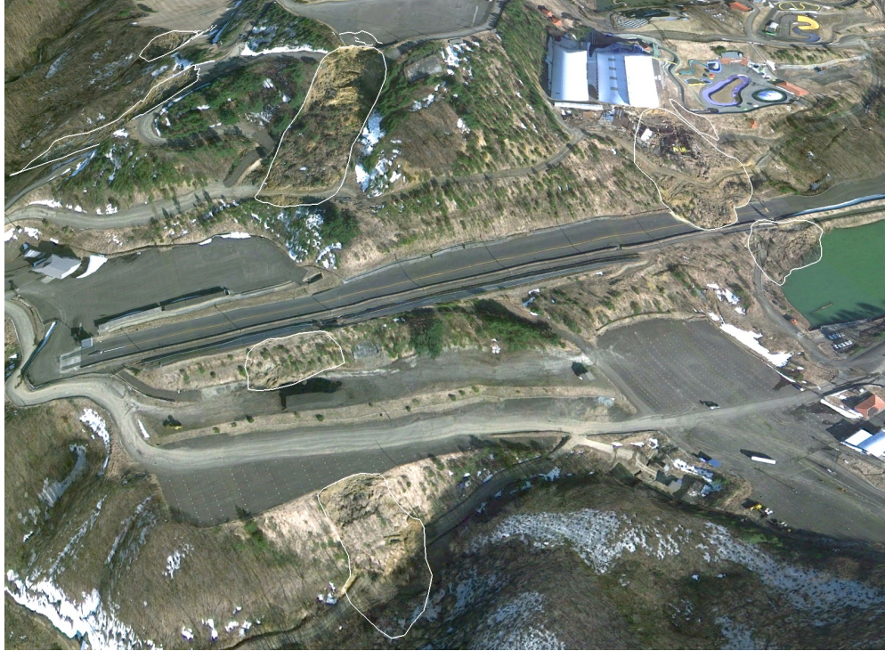
Figure 2.11 Example anthropogenically modified landslides in the foothills of the Ou Mountains west of Sendai, Japan. Landslide bodies outlined in white. For all landslides the source region abuts either a roadway or parking lot, with some landslides failing entirely in anthropogenic fill deposits.
