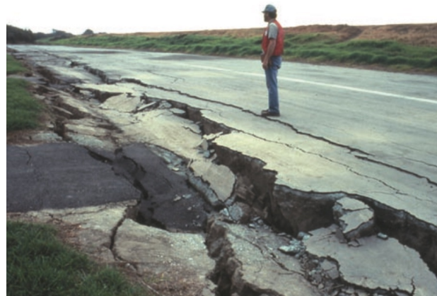
Figure 2.10 Simplified diagram (left) and an example Lateral Spread. Located in modified landscapes (e.g., levees, irrigated fields, and golf courses as in the above). Often extensive, with complex boundaries and movement. Visible deformation correlated with slope or proximity to a free face. Located in near-flat terrain, sometimes transitioning into flows when steep topography is located directly below source zone. Figure from Highland and Bobrowsky (2008), based on Cruden and Varnes (1996), photograph by Steve Ellen.
