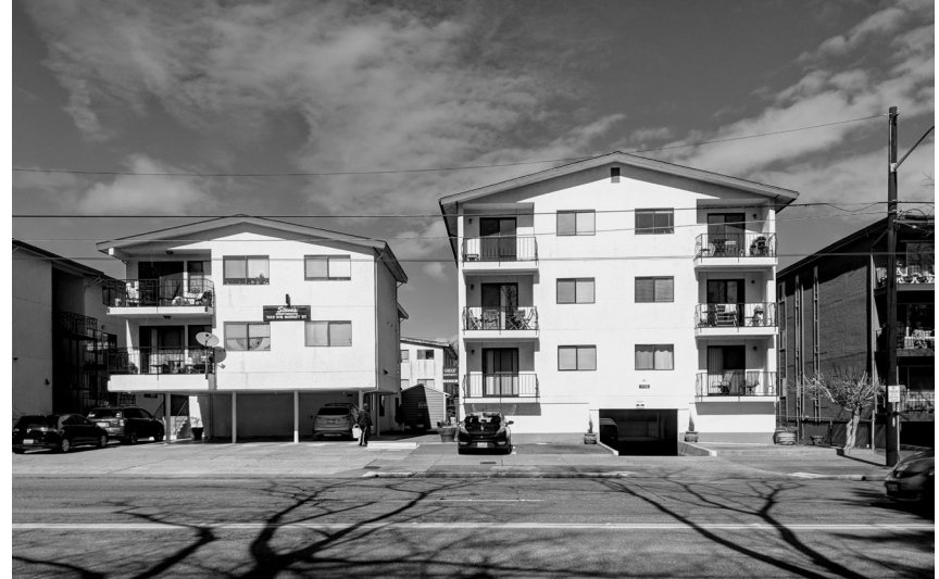
Fig. 85 - Low Rise Apartment Eastern Ballard, Photo
