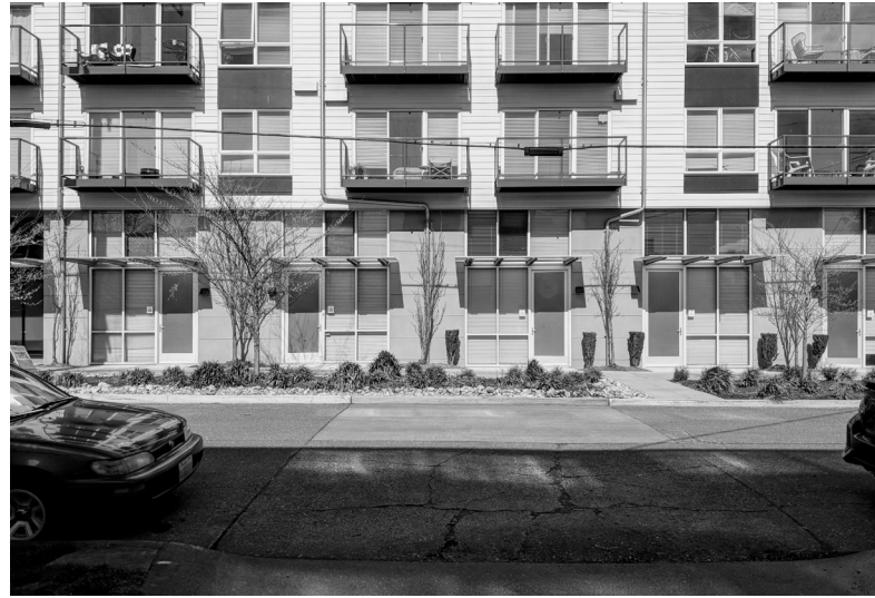
Fig. 89 - Apartment Eastern Ballard, Photo
