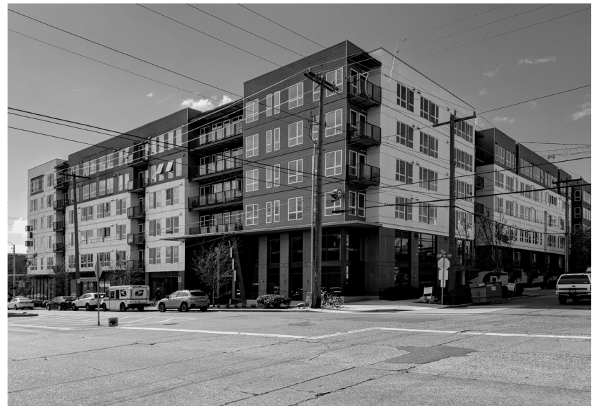
Fig. 87 - 5-over-2 Eastern Ballard, Photo
