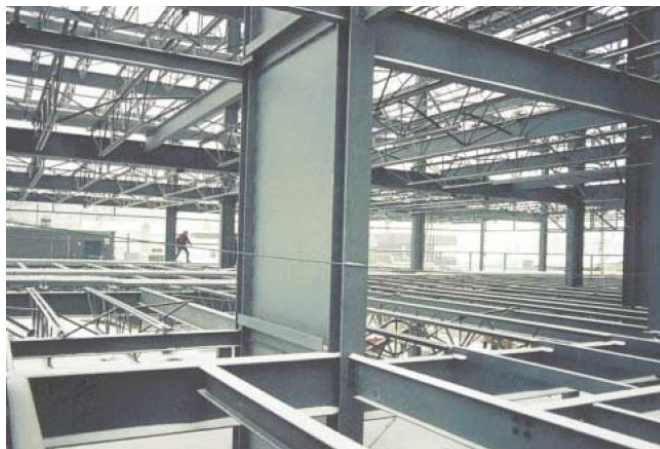
Figure 1.1: SPSW During Construction
