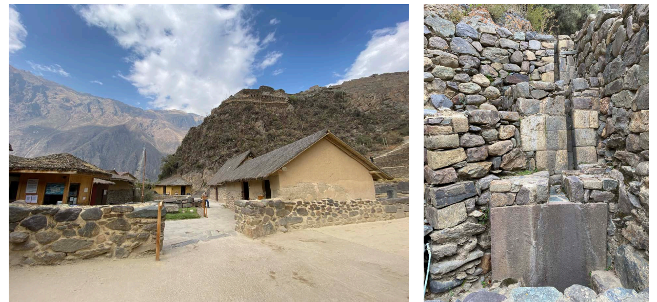
fig. 68 (top), Stone, adobe, and thatched roof building, Ollantaytambo, September 2024 image by author
