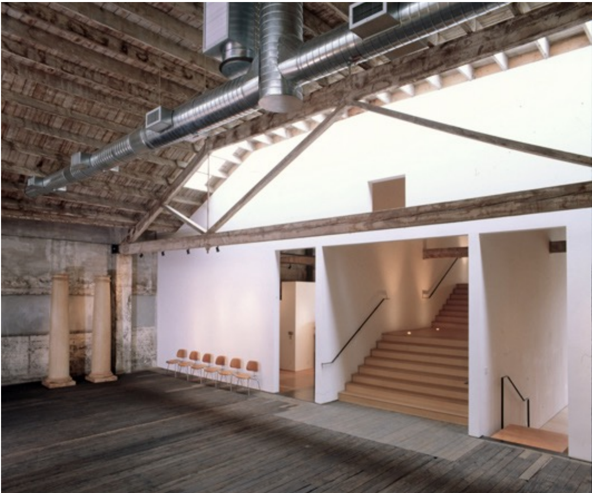
Figure 1 - Suyama Space gallery, between retail storefront and architecture studios
