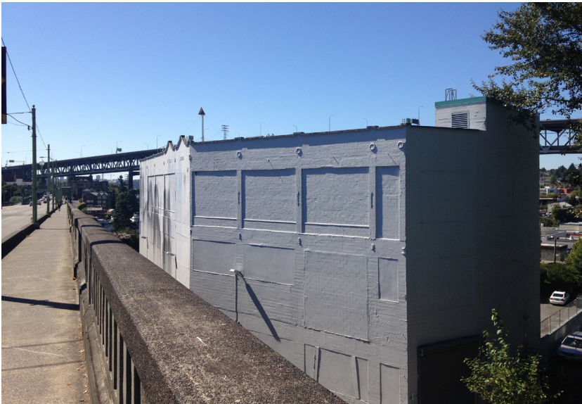
Figure 4.14 East Facade from Bridge with I-5 bridge visible beyond
