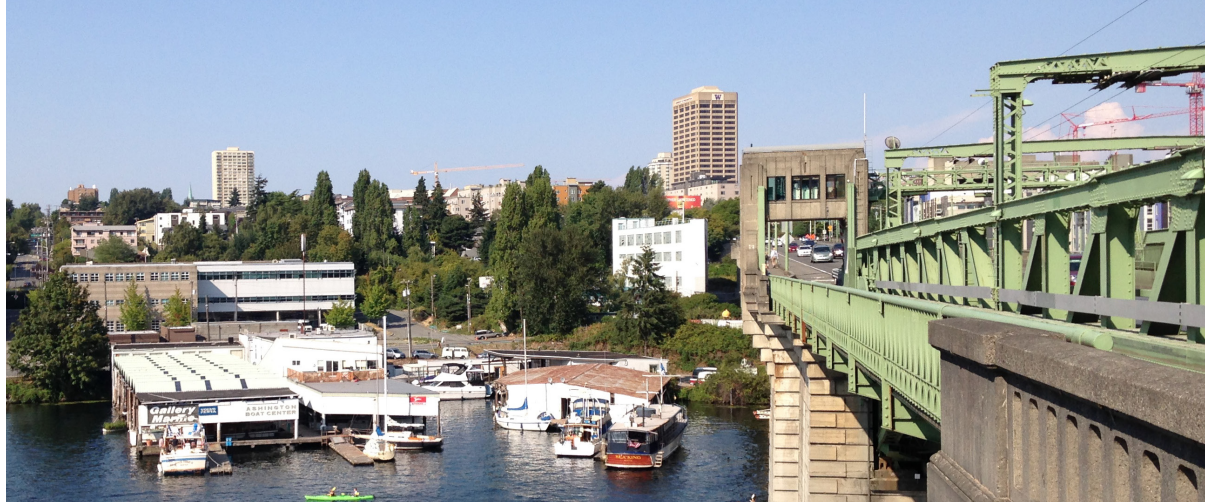
University Bridge - el. 90'
