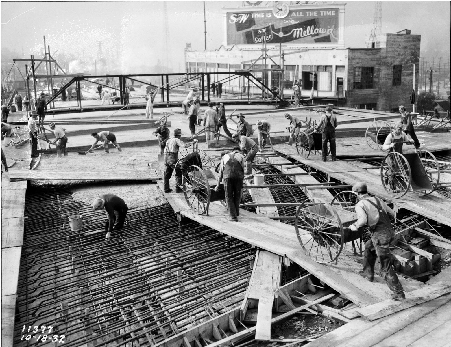
Figure 4.19 - 1932: Bridge Rebuild with Exterior Sidewalk Visible
