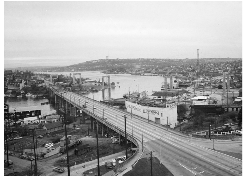
Figure 4.21 - 1959: I-5 Bridge Under Construction
