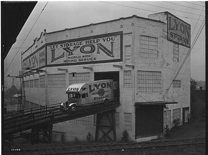
Figure 4.20 - 1937: Building as Billboard
