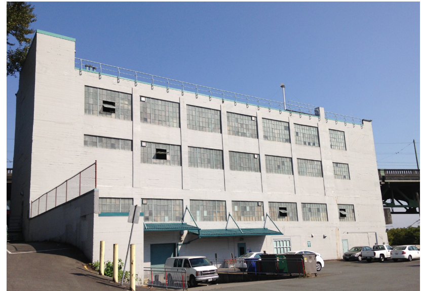
Figure 4.15 West facade with original windows
