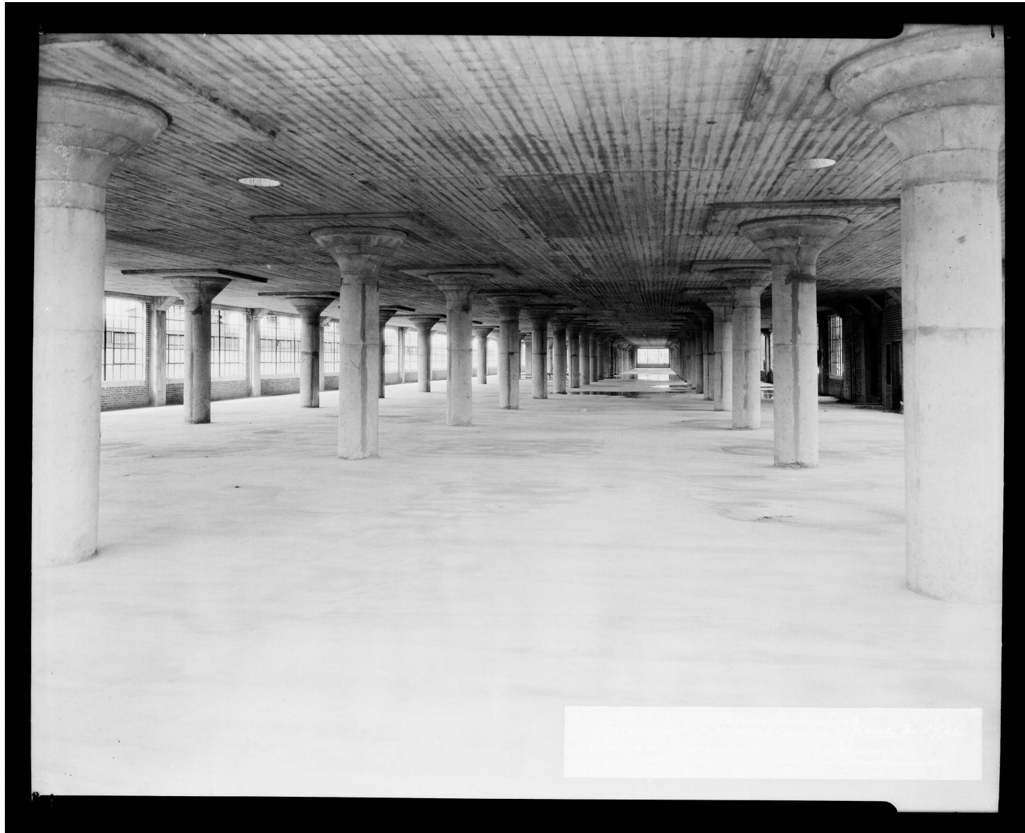
Figure 27 - Interior of production building during construction
