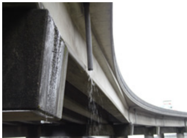
Figure 2.10) Conditions under the Existing SR 520 Structure
