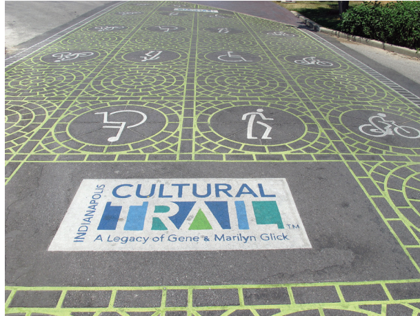
Figure 24. Duratherm intersection treatment, created with a thermoplastic material inlaid in the asphalt. (Creative Commons: Jun Wang)
