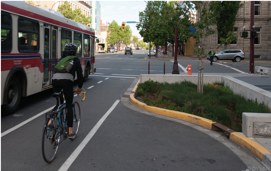
Figure 12. Complete Streets enhancements can include intersection improvements such as bulbouts, green stormwater and bicycle infrastructure shown above in Victoria, BC (Creative Commons: Dylan Passmore)
