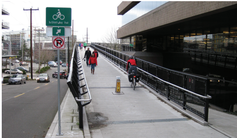
Figure 17. West Thomas St Pedestrian and Bicycle Overpass north (Queen Anne) entrance (Schwindeller 2014)
