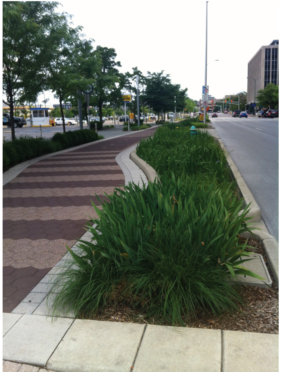
Figure 26. Stormwater planter showing curb cut (Credit: Indianapolis Cultural Trail)
