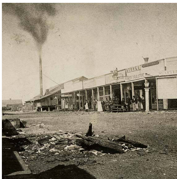
(a) Looking West, 1873
