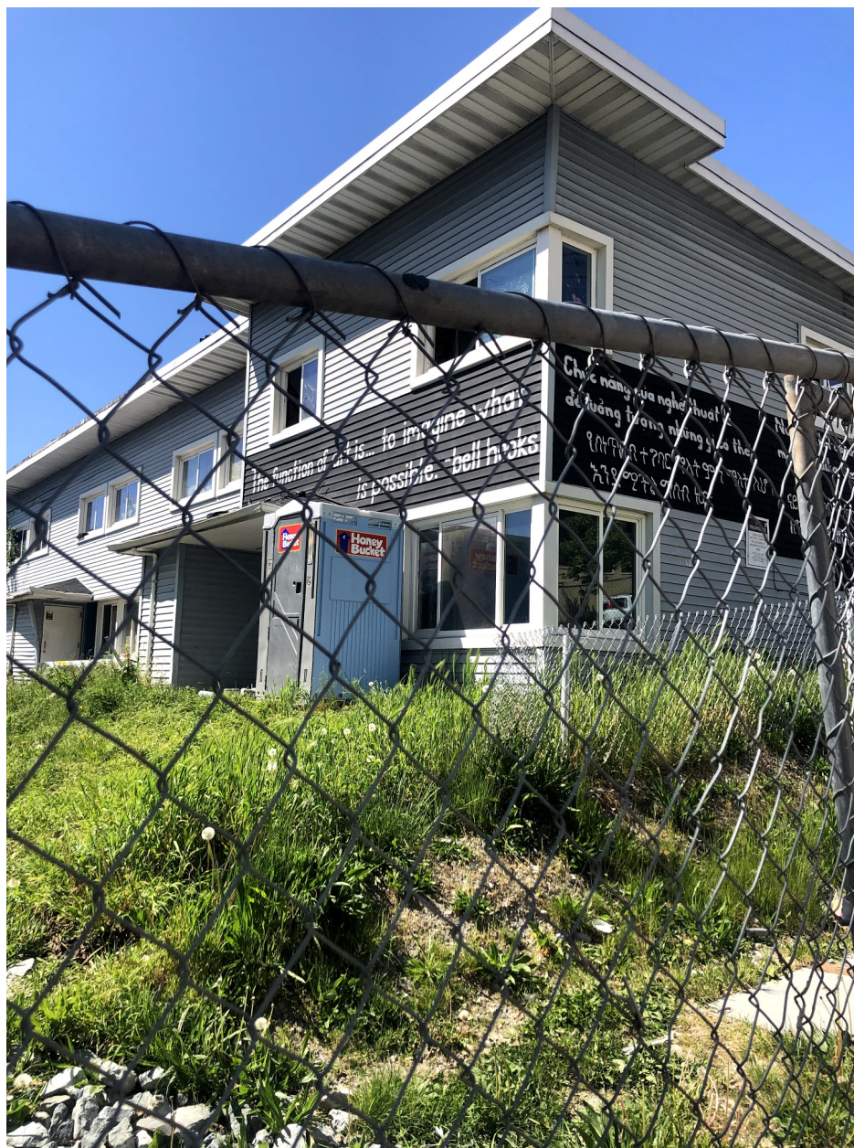
Figure 1: Rowhouses at Yesler Terrace before Demolition, May 2019
