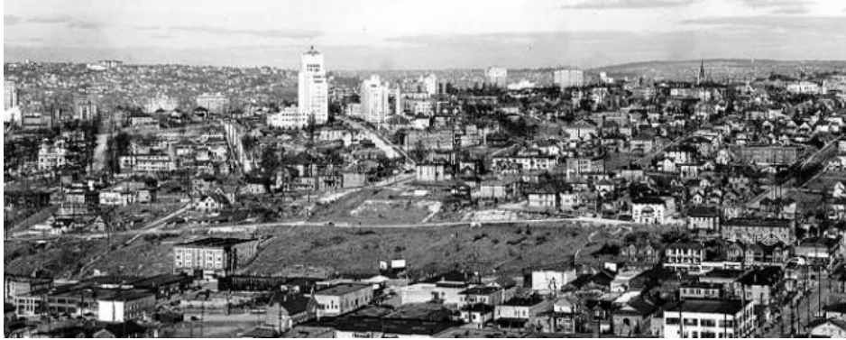
(a) Profanity Hill before Demolition, 1940
