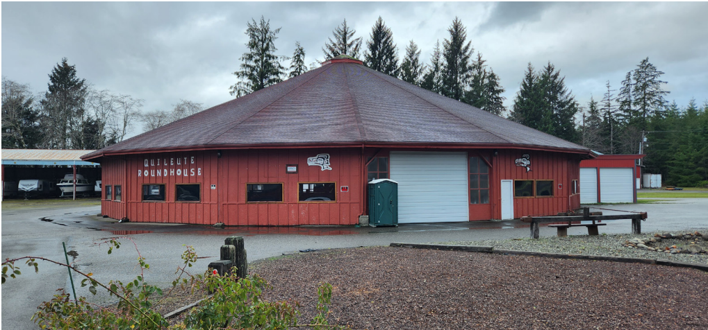
Figure 3: Main, East Elevation [Image source: Author, Jan. 2023]
