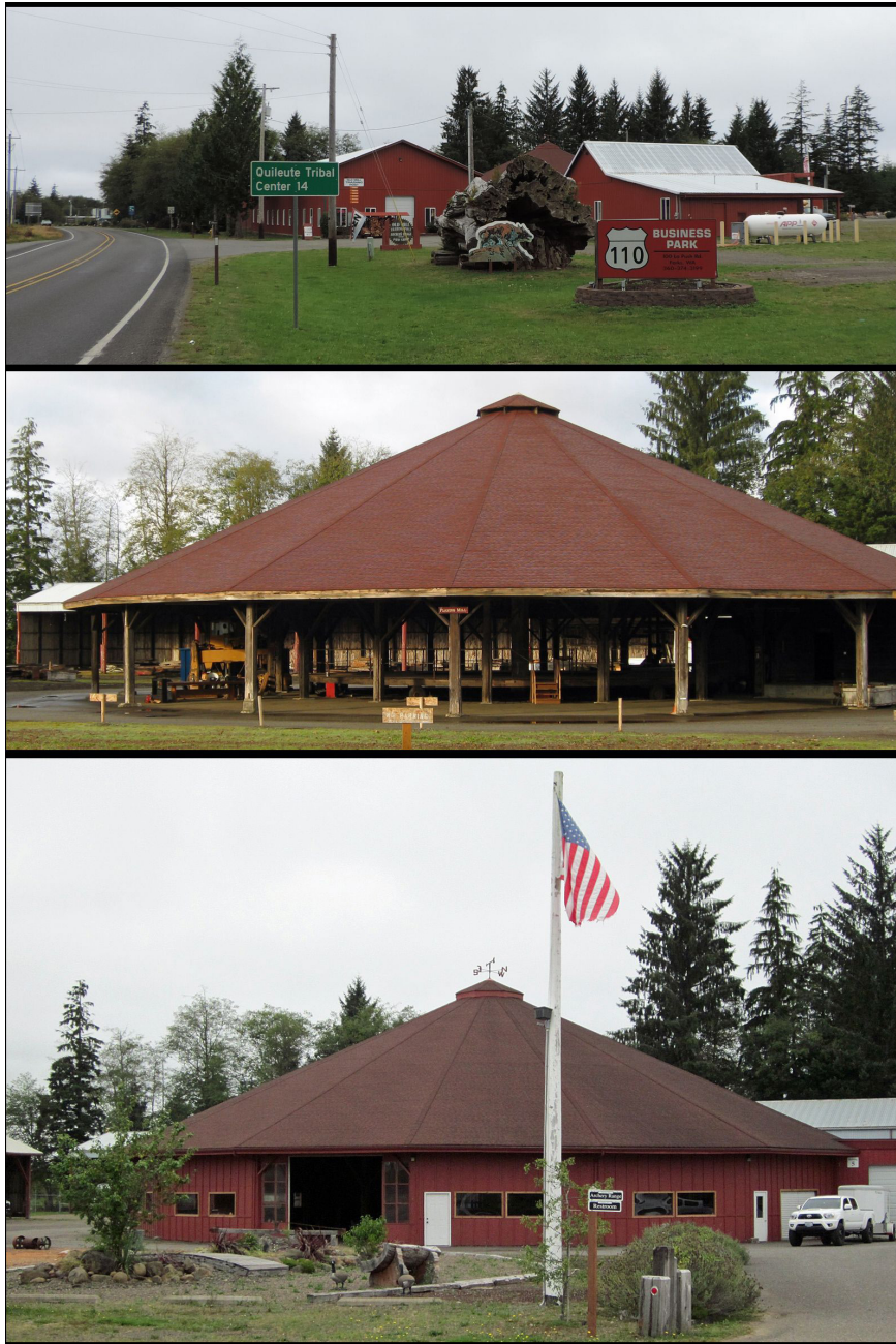
Figure 29: Before and after the Round Shed was enclosed. [Image Source: Pinterest]
