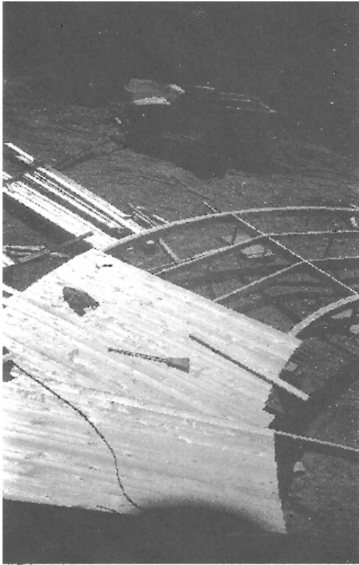
Figure 22: Constructing the Big Wheel, 1960. [Image Source: Tom Rosmond.]
