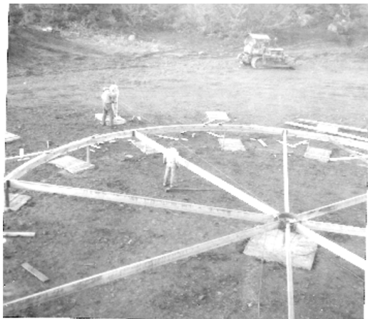
Figure 23: Laying deck on wheel, 1960. [Image Source: Tom Rosmond.]
