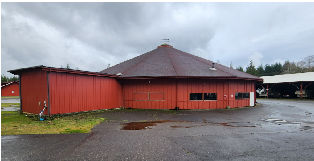
Figure 4: West Elevation [Image source: Author, Jan. 2023]
