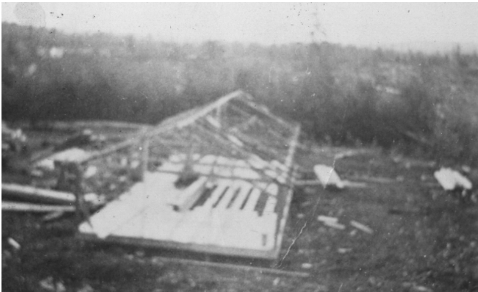
Figure 19: Framing the Sawmill Building, 1946. [Image Source: Tom Rosmond.]
