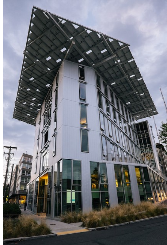
Fig.1 The Bullitt Center performing the process of night flushing
