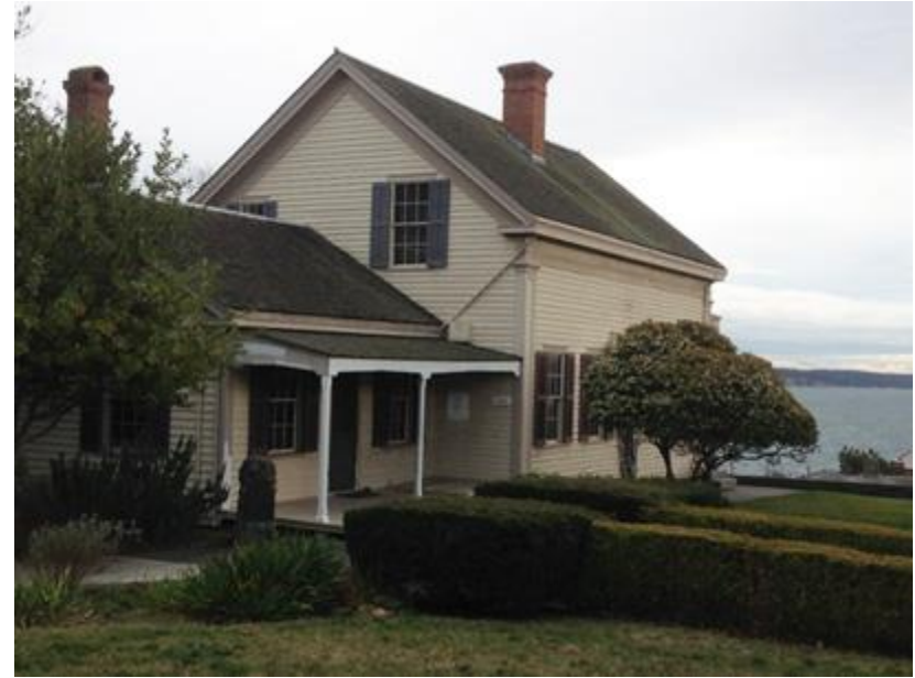
Figure 4.20. Kitchen porch and English Boxwood borders and lawn in the foreground in the southwest view. February 5, 2016.
