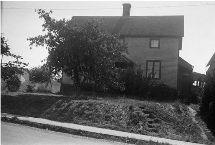
Figure 2.21. In this north view of the Haller property, the front yard sloped down to the boardwalk on Front Street. On the photo right, a dirt path leading to the side entrance, the conservatory is visible in the rear, and a cinema stands on the right picture edge. The yard included some grass, a tree and ornamentals around the foundation. June 22, 1948. Historic American Building Survey. HABS WASH. 15. COUP. 6—1
