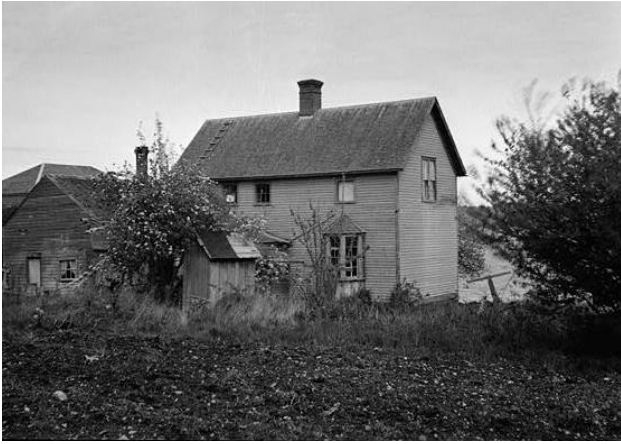
Figure 2.23. Southeast view of the Haller property backyard. The south bay window offered views of the private backyard. The neglected backyard included ornamental trees and shrubs. June 22, 1948. Historic American Building Survey. HABS WASH. COUP. 6—3
