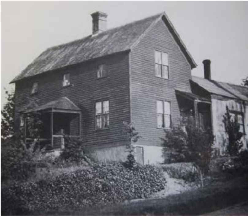
Figure 2.26. In the northwest view a dirt path leads to front entrance. The yard included groundcover, possibly English Ivy, grass and shrubs. The conservatory and store had been removed. Post 1954. University of Washington Libraries, Special Collections Division.
