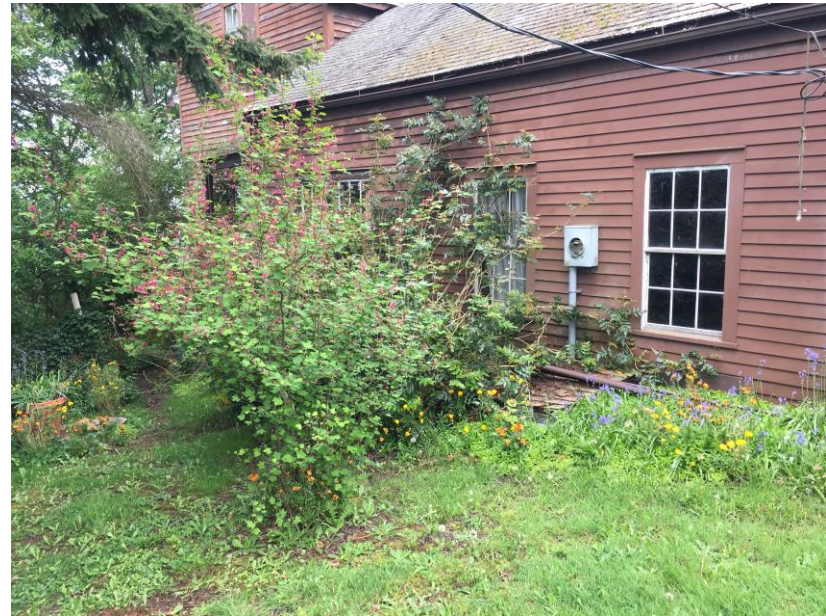
Figure 2.39. West side view of the overgrown side yard. Early photographs show a conservatory was once located on the west wall. March 2016.
