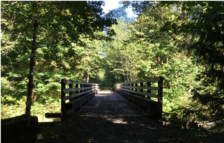
Figure 34: Bridge with guardrails
