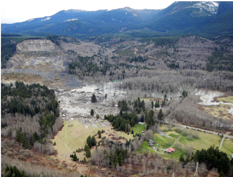
Figure 20: View north of 2014 landslide
