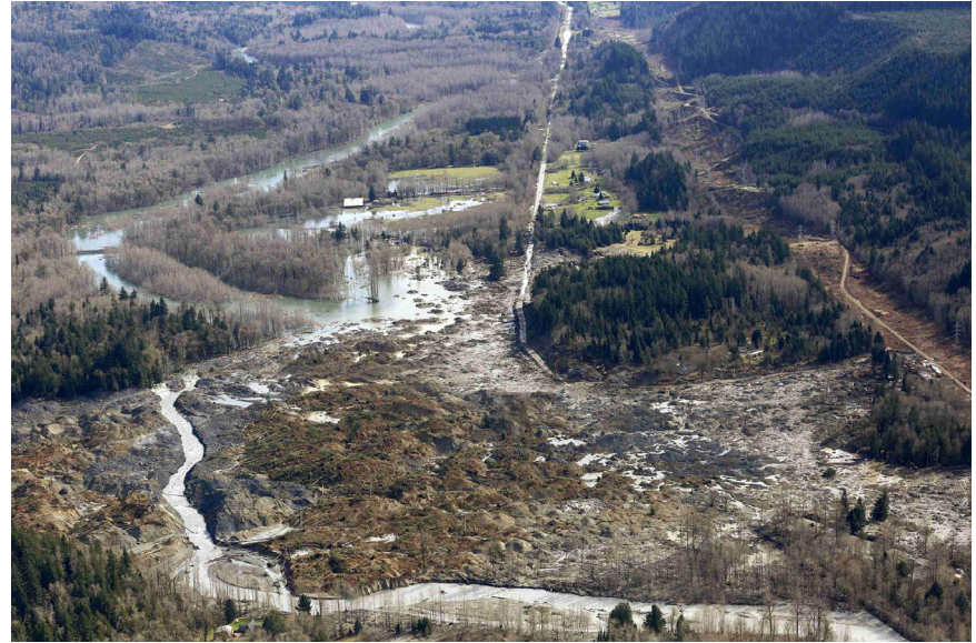
Figure 33: Trail (and highway) destroyed in 2014 landslide
