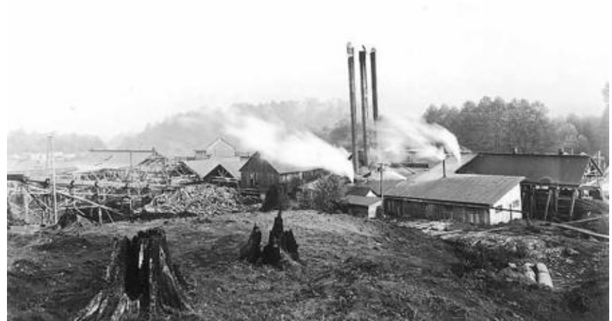
Figure 30: Old Fortson Mill
