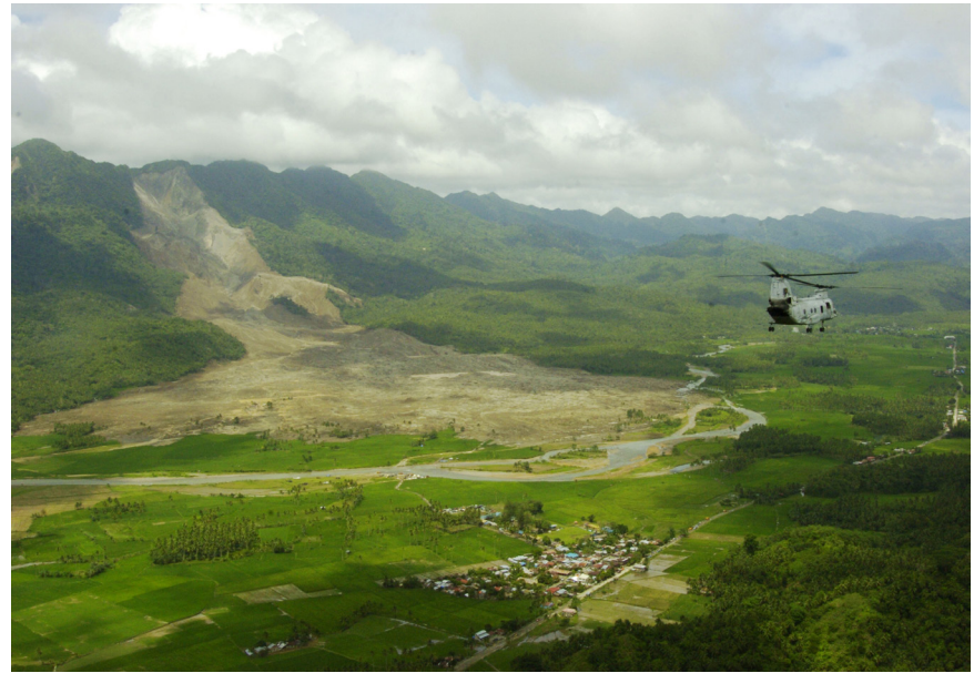
Figure 3: Former village of Guinsaugon after landslide
