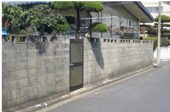
Figure 16. Current House Brick Wall
