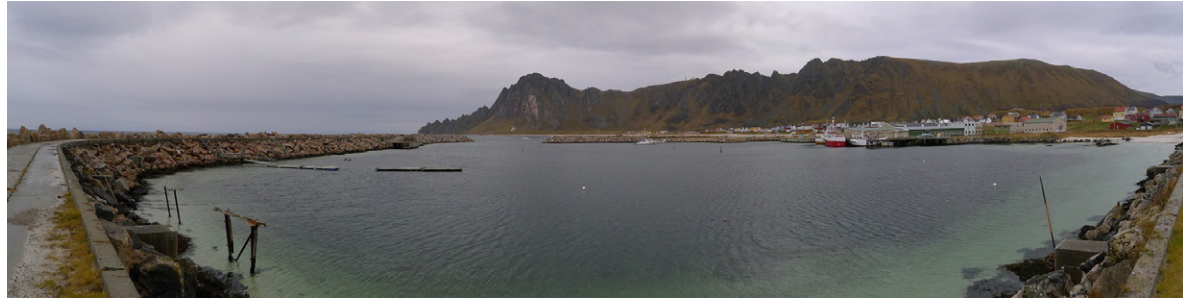
fig. 158 View of Bleik Harbor from the seawall.
