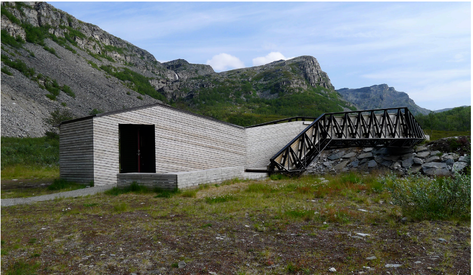
fig. 33 Service building and prefabricated steel and wood bridge, Lillefjord. Havøysund NTR.
