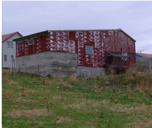
fig. 165 A weathered out-building, Bleik.
