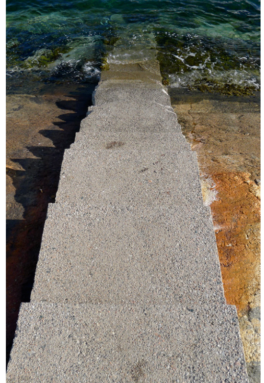
fig. 26 Stairs into the water.
