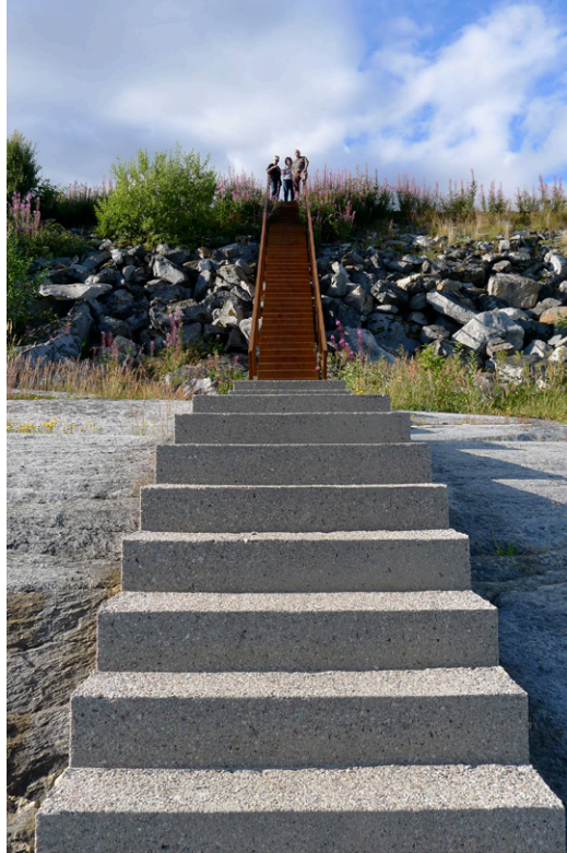
fig. 25 A path of concrete and steel.
