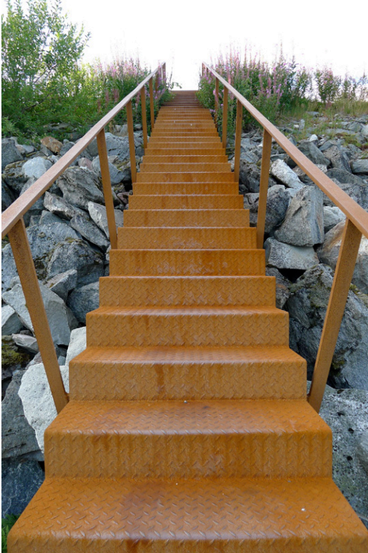
fig. 24 Looking up the top of the stairs.
