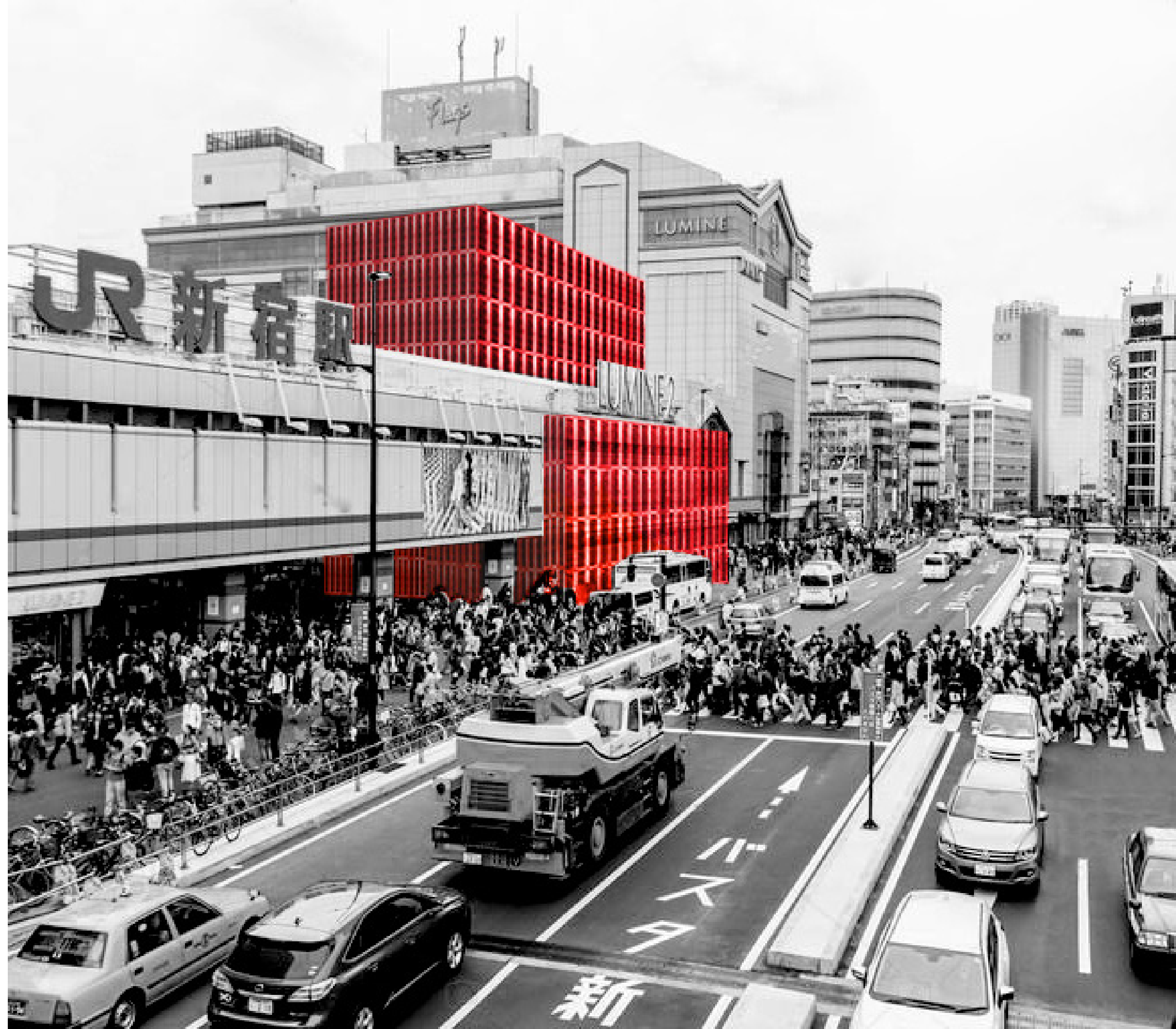
Figure 54 Data center located at Shinjuku Station entrance.
