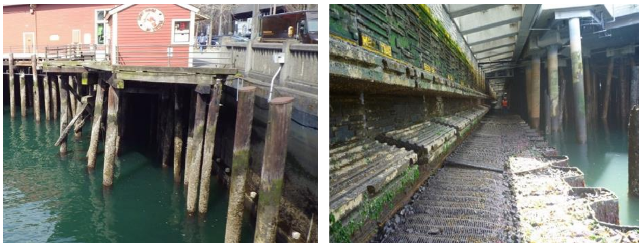
Figure 1.1. Photographs of Seattle's seawall, with enhancements, before and after reconstruction.
