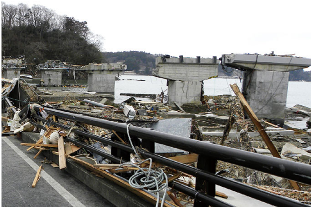
(a) Utatsu Ohashi Bridge, Japan (2011)
