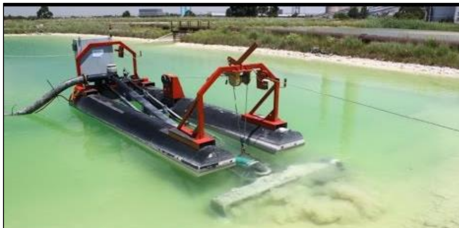
Figure 5-2. S.A.M.E. auger dredging, Australia
