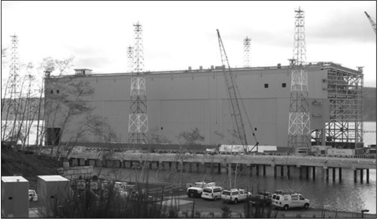
Figure 6-11 Structural Steel Project (Source: Daily Journal of Commerce, Seattle, WA January 23, 2017)
