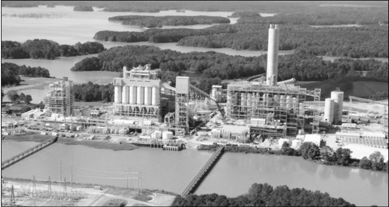
Figure 6-7 Piping Project Power Plant
