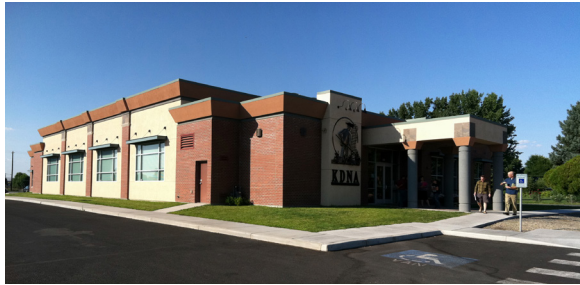
Figure 17. Exterior of NW.C.E.C.
