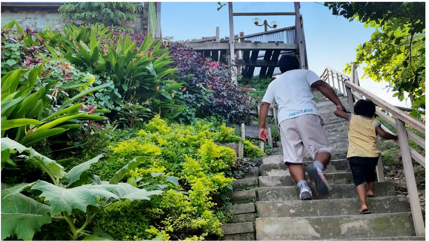
1 year after construction
