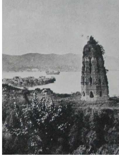
Picture of Leifeng Pagoda from the Republican Period before it collapsed. Photo from Zhang Daqing, Jiang Bingxian, Xihu jiuzong (Hangzhou: Zhejiang renmin chubanshe, 1985), 20.
