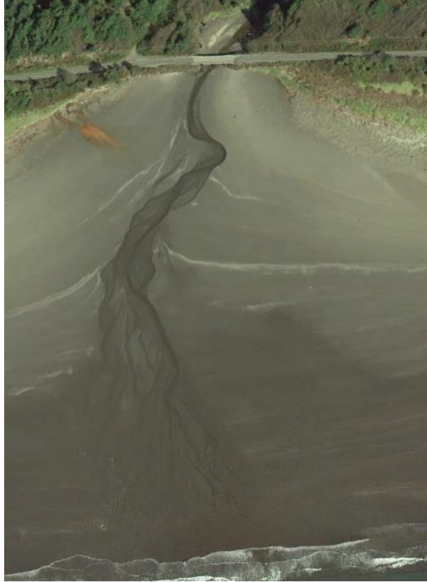
Figure 6-1: Wreck Creek Bridge: 47° 17' 4.54"N, 124° 14' 1.51"W (Google Earth™)
