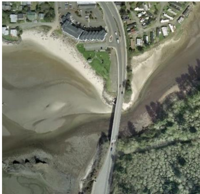
Figure 6-5: Schooner Creek Bridge 44° 55' 32.55" N, 124° 0' 49.87" W (Google Earth°)
