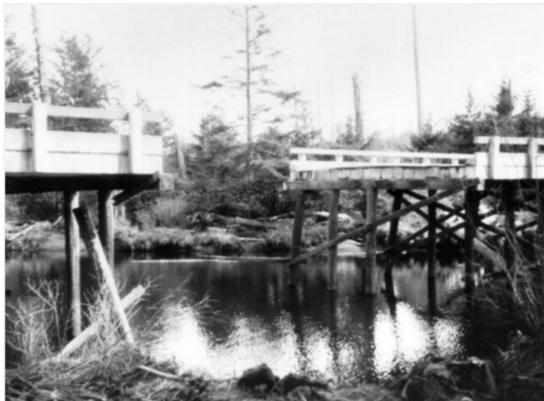
Figure 6-3: Joe Creek Bridge Damage from 1964 Alaskan Earthquake and Subsequent Tsunami (reprinted from TsuInfo Alert, [February, 2014])
