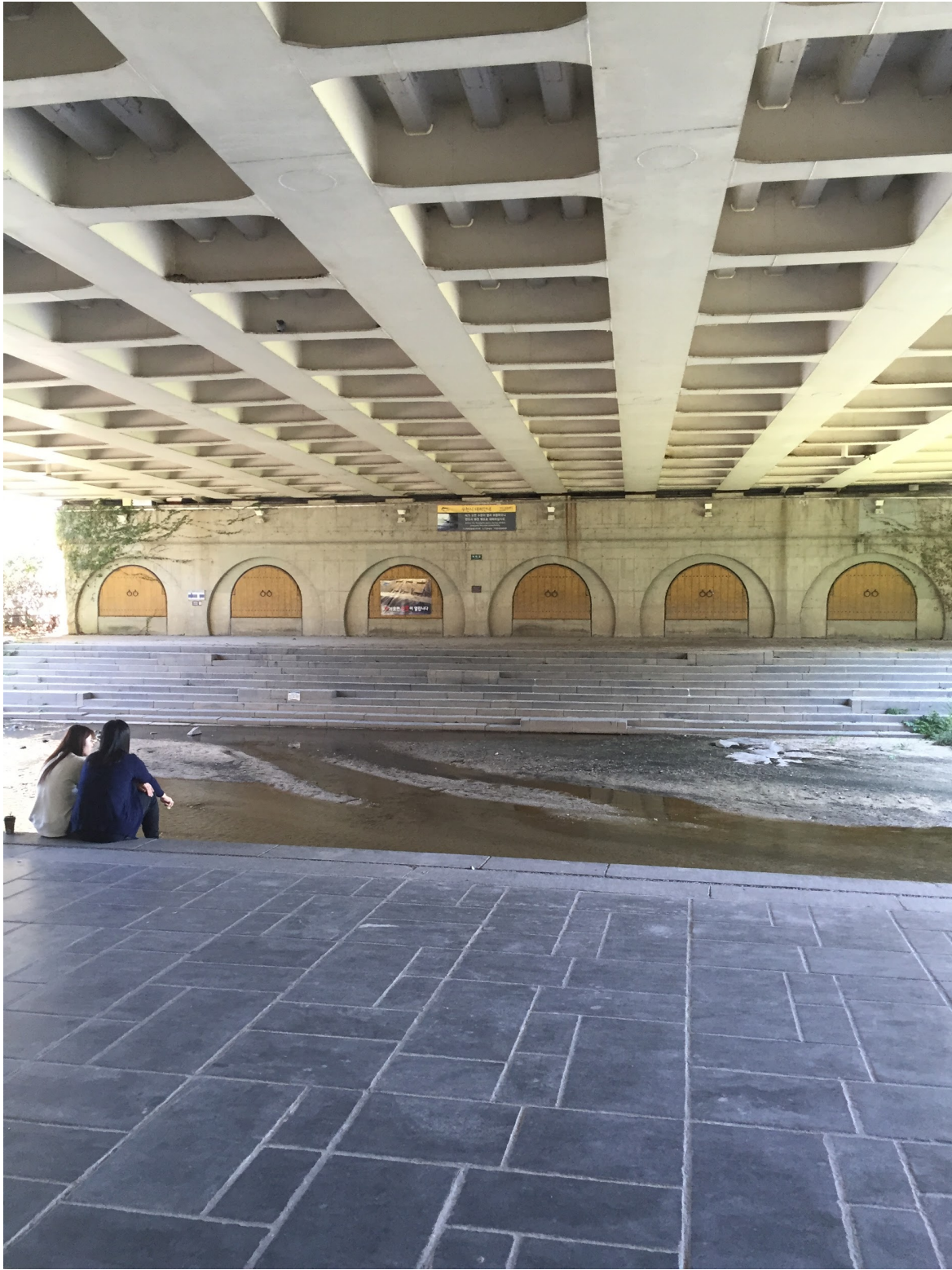
Figure 2: Cheonggyecheon floodgates under Muhak bridge (“Muhakgyo”)
