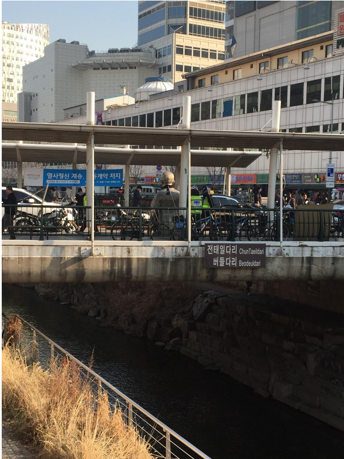
Fig. 50: Chun Tae-il Bridge/ Beodeuldari Bridge
