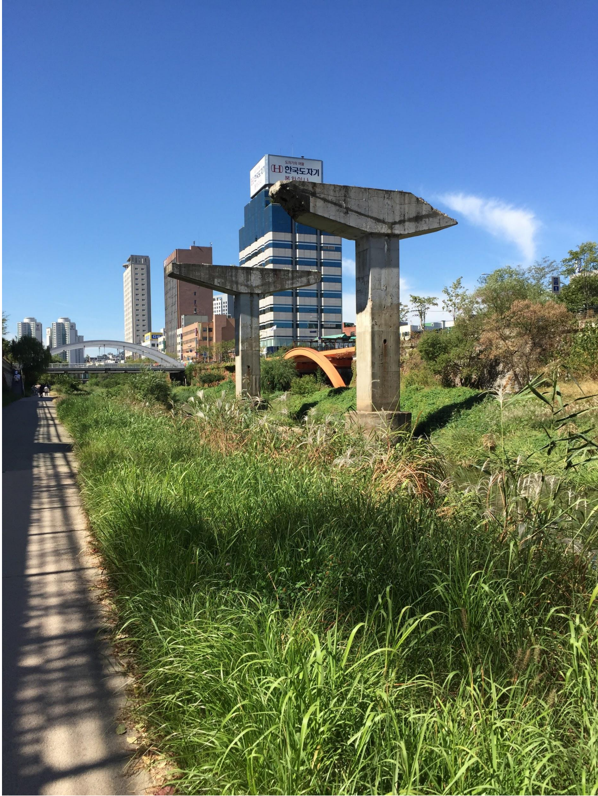
Fig. 57: Remains of the columns of the highway ramp
