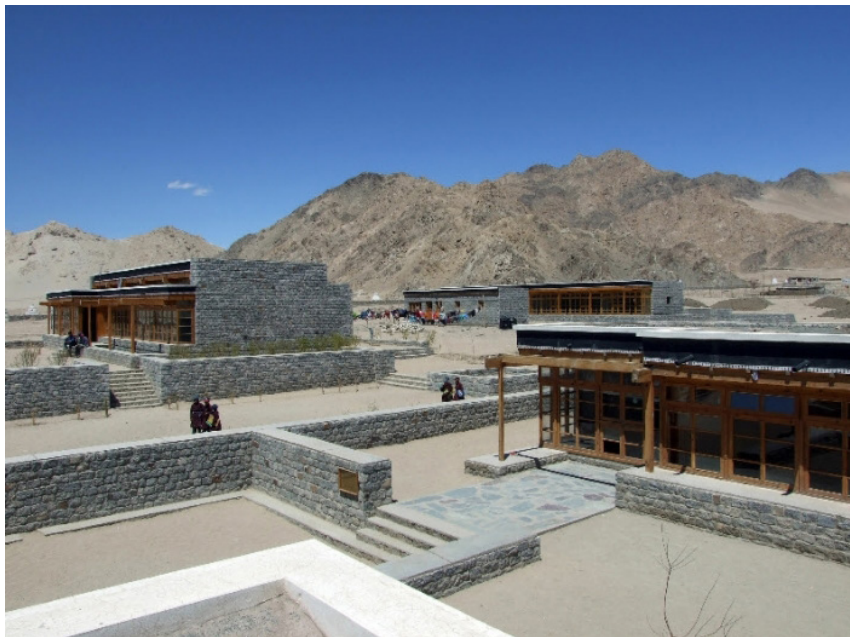
Solid granite blocks used for the outer wall come from stone found on or adjacent to the site. Inner walls are made from local mud brick,
