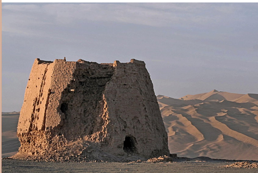
The rammed earth building remains on the Silk Route.
