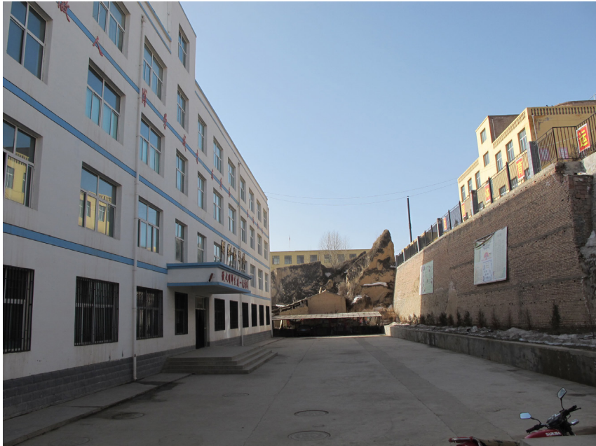
The site was divided in two parts, one is leveled with the street, the other part is raised up to 20 feet above with a huge retaining wall.
