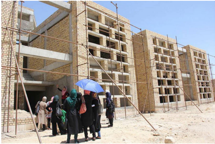
The Gohar Khatoun Girl's school during construction.
