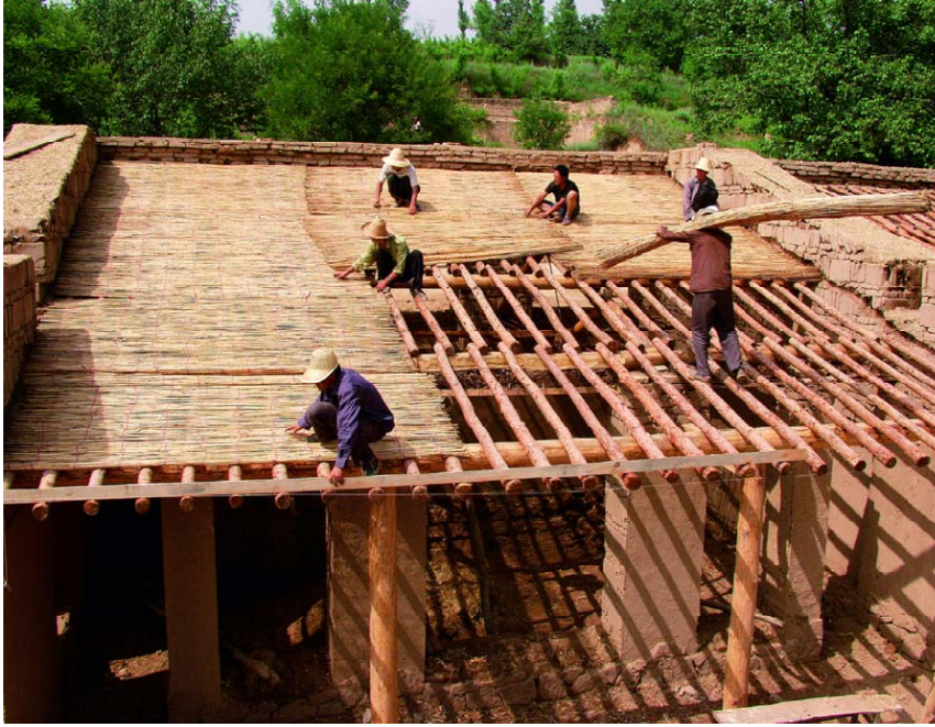
Local building materials and low technique construction.
