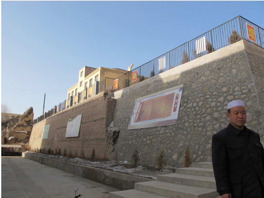
The huge retaining wall.
