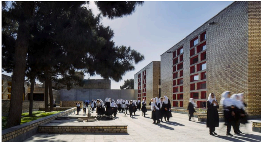
In this school all of the landscaping is irrigated using biologically treated wastewater.
