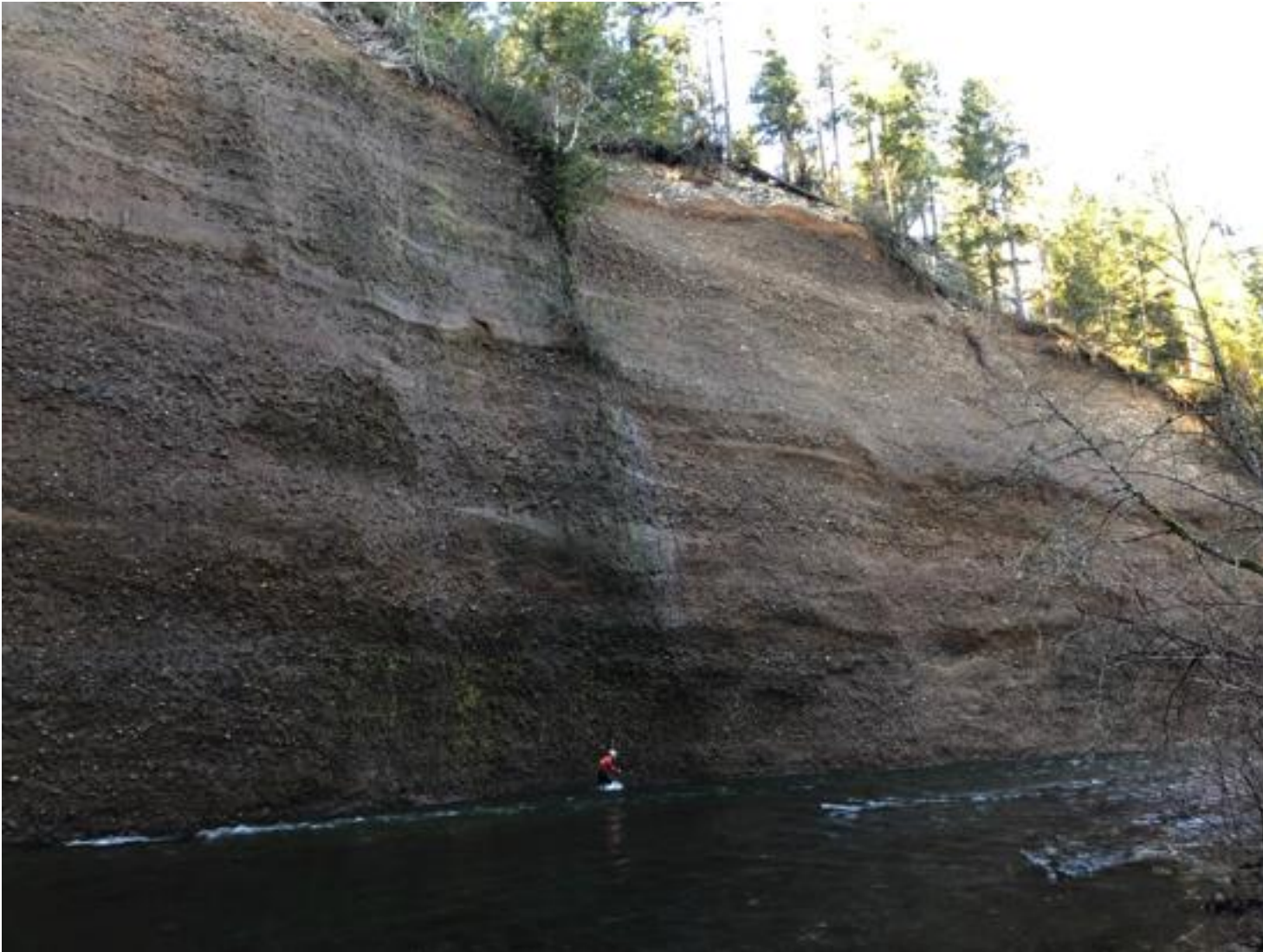
Figure 3. Eroding bluff of interest at rkm 33.4 characterized for cumulative grainsize distributions using image analysis. Maximum bluff height is 33.4 m. Photo is taken from the right bank. River is flowing from left to right.
