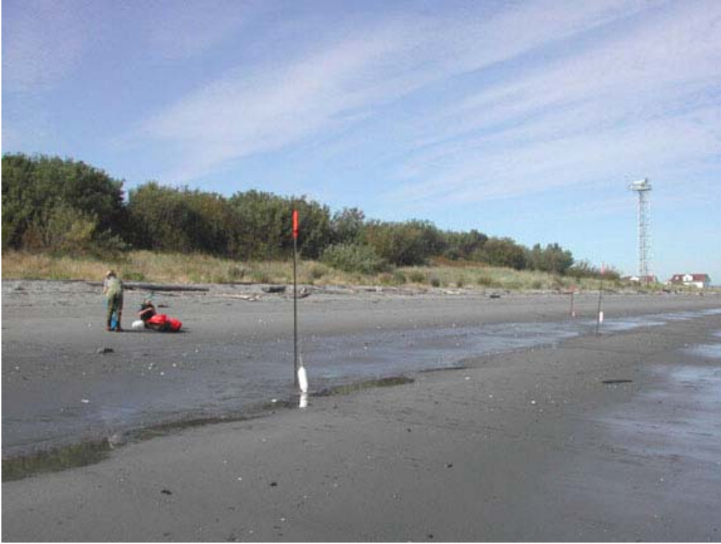
Figure 3. Installation of enclosure net and video mounting poles at West Point during low tide the day before sampling.
