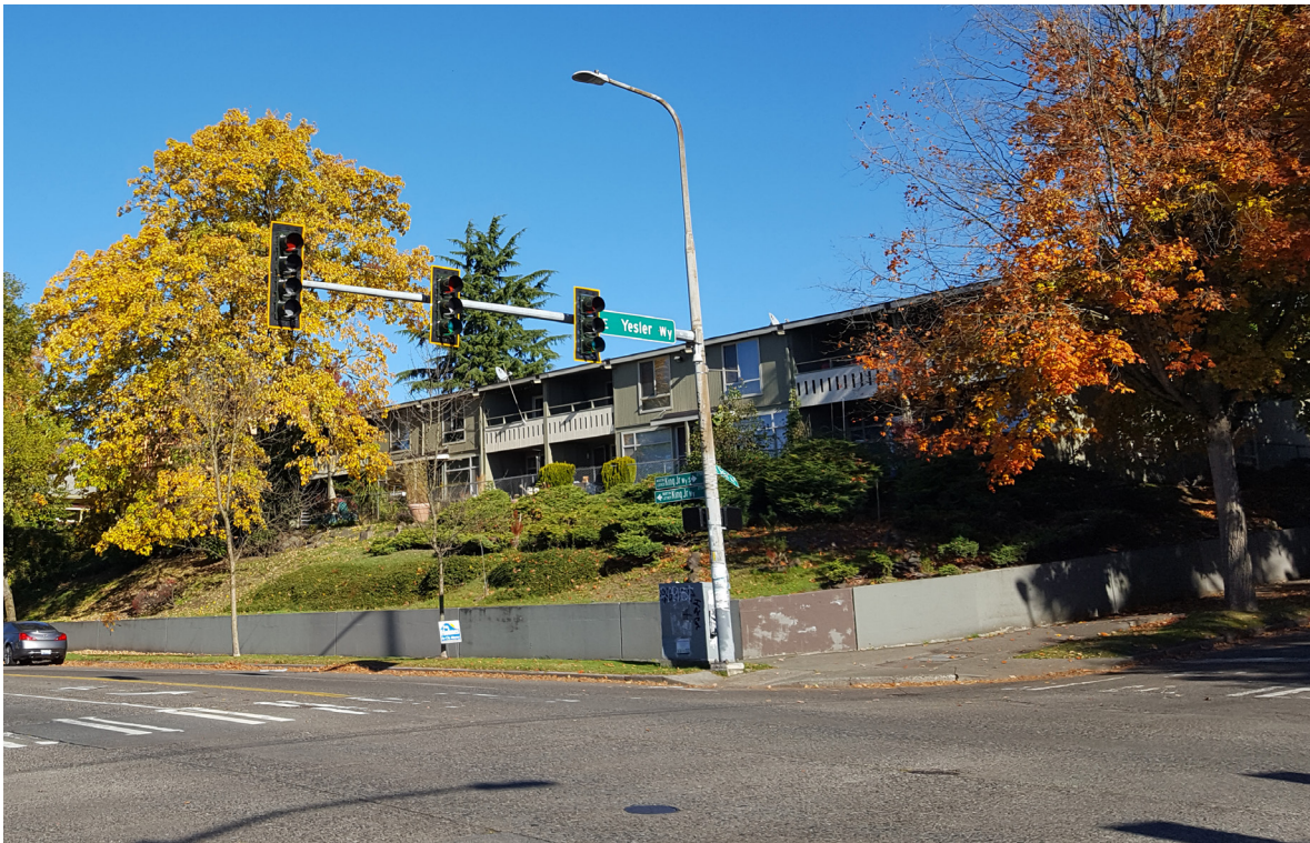
Figure 33 - The project site, showing the retaining wall and neighboring building
