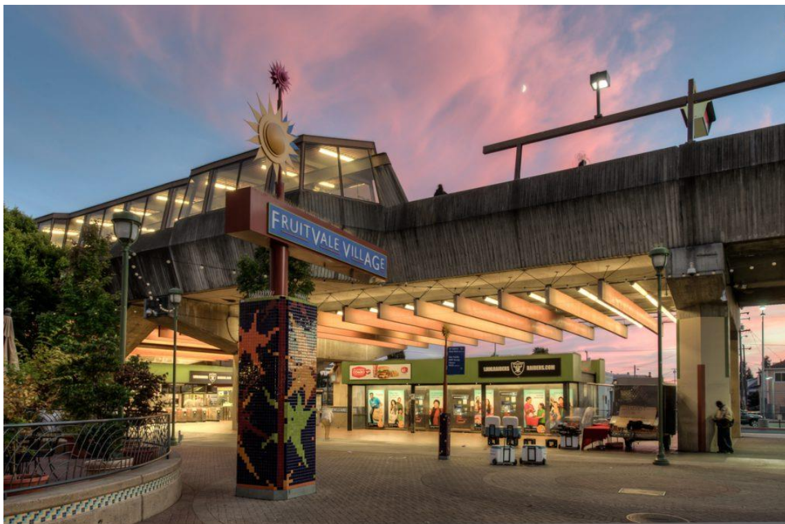
Figure 4.11. The BART station at Fruitvale Village (PGA design).
