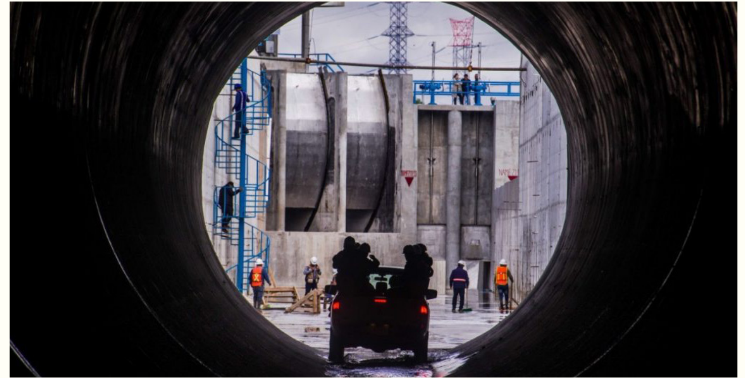
Construction of the 'Western Outlet' Fig.1 Cuartoscuro, 2022.
