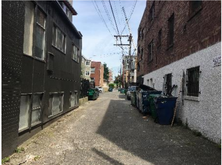
Figure 5.21. Spilling Over into the Right of Way
