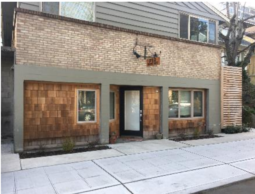
Figure 6.11. Reclamation Starts from the Garage at 712 Summit Ave E
