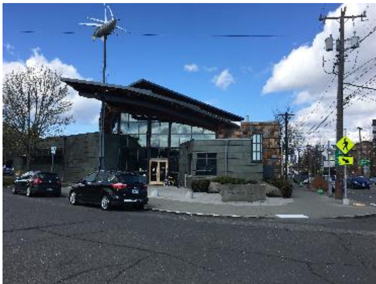
Figure 5.12. Beacon Hill: Library and Light Rail
