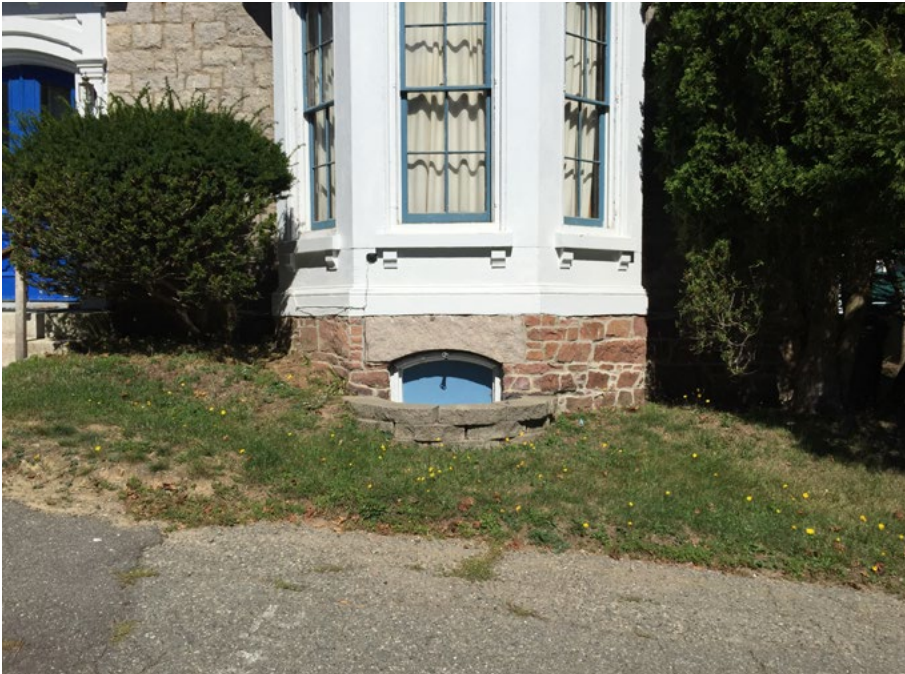
12. Granite foundation, Eastport ME
