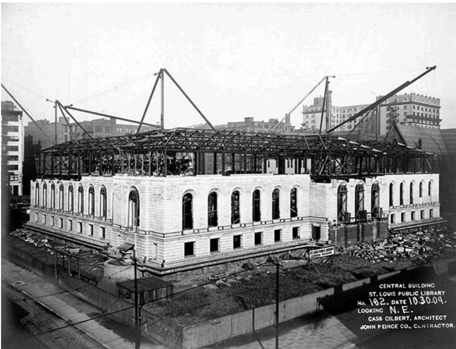
13. Maine Granite making up the exterior of the St. Louis Public Library, MO
