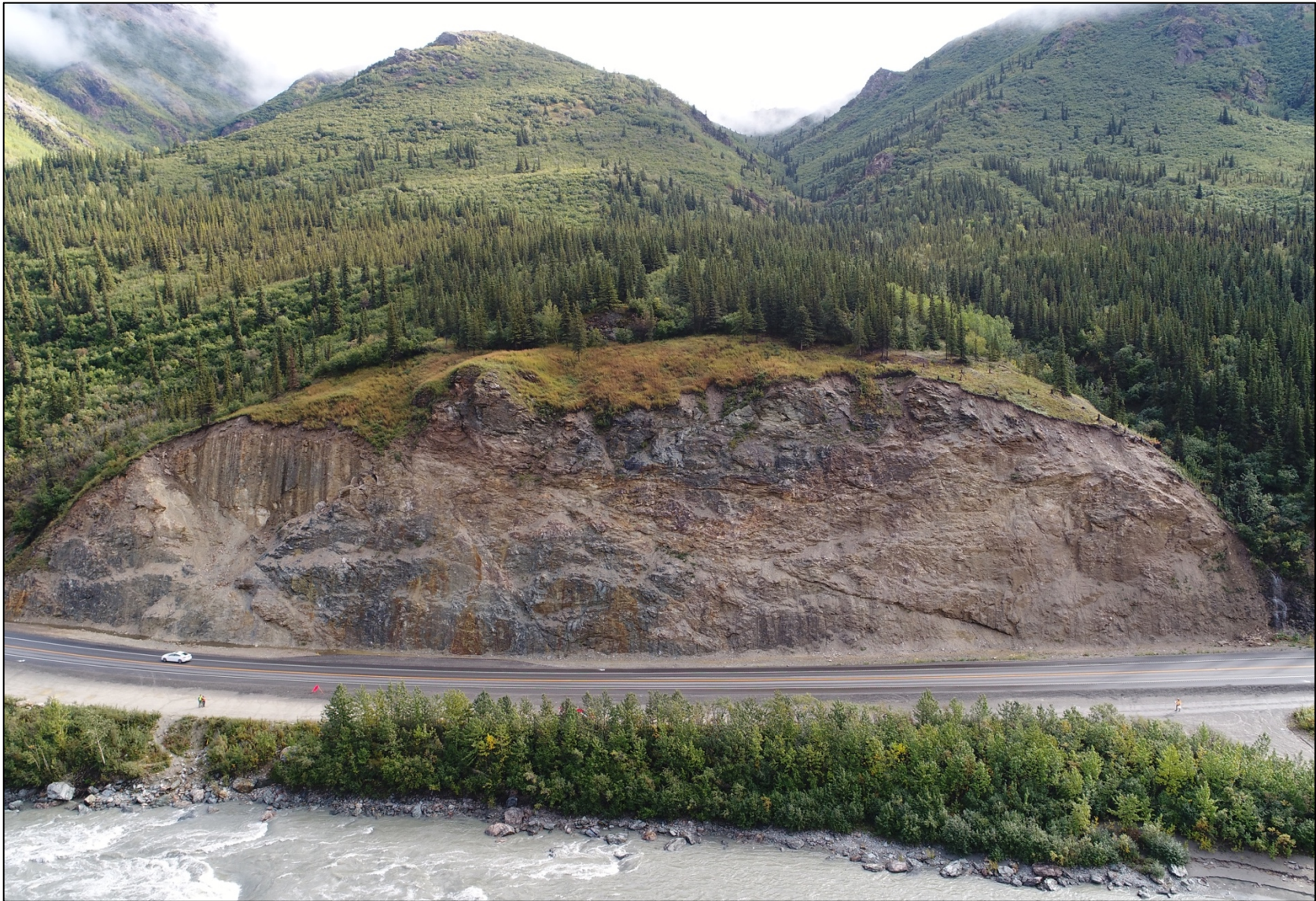
Figure 7: Aerial photo taken in August 2018, of the study slope at MP 241 on the George Parks Highway near Glitter Gulch, Alaska. The image was captured with a DJI Phantom 4 drone flown by Jake Dafni. North is to the left; Sugar Loaf Mountain is in the distance and the Nenana River is in the foreground. Quartzite dominated regions of the outcrop present as grey while more micaceous regions appear brown in this image.
