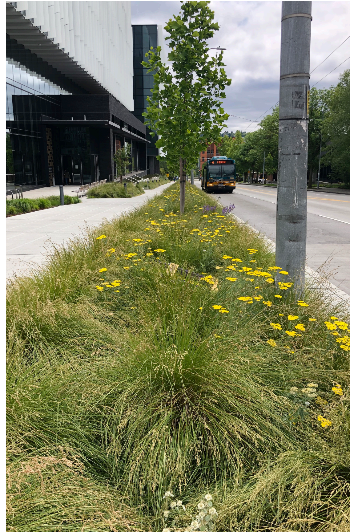
Figure 6-1. The understory of street trees adding diversity and acting as green stormwater infrastructure
