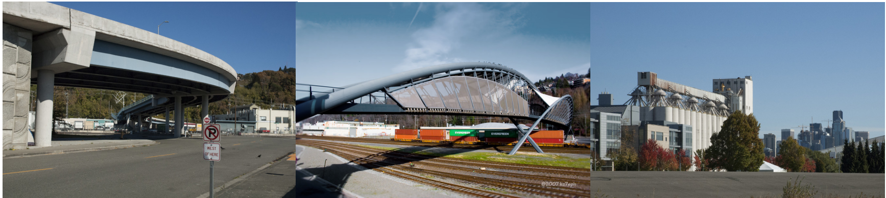
Figure 27: Industry and infrastructure surround and shape the site.
